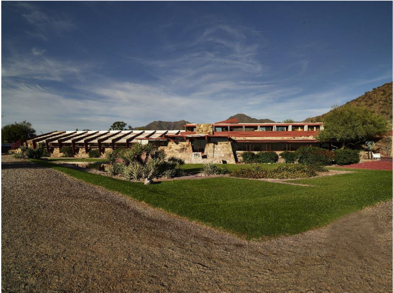
Taliesin West and Jester-Pfeiffer House
