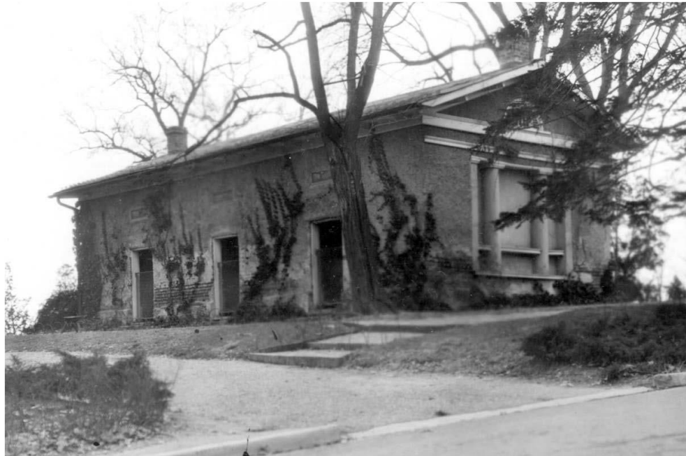
Figure 29 – South Dependency NW Corner in 1938, looking SE (NPS ARHO Collections)
