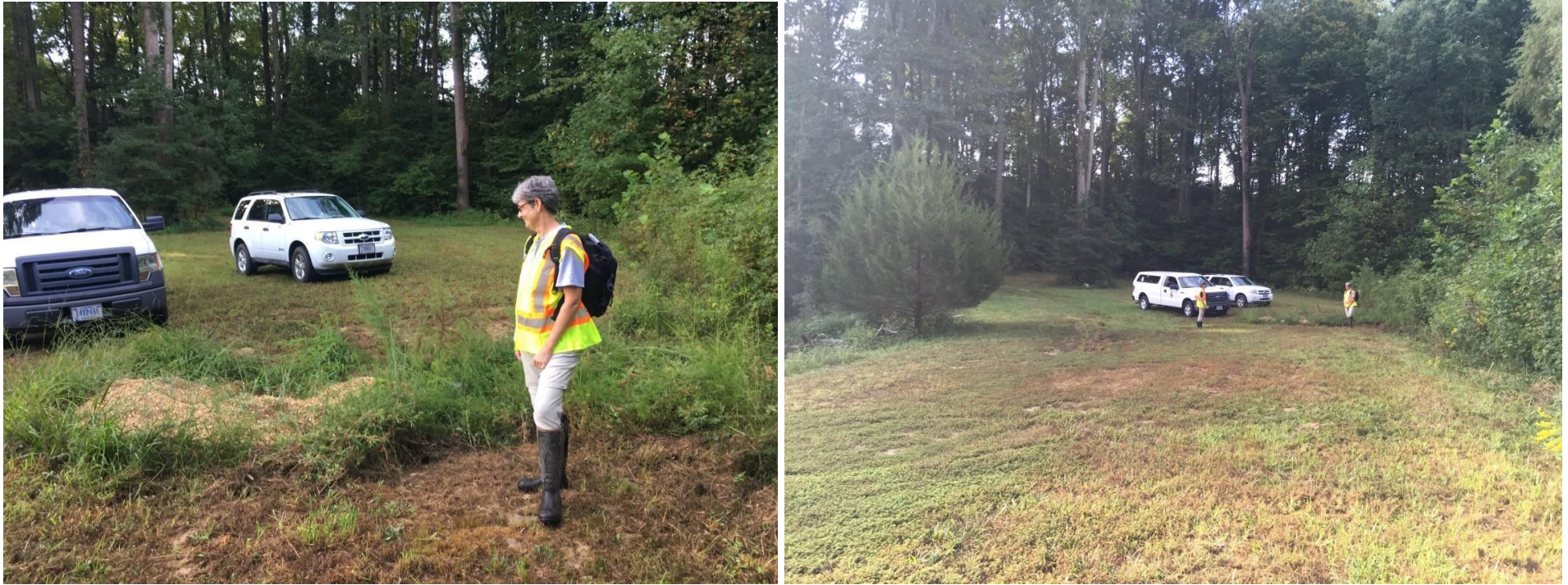
Figure 6: Filled Sinkhole on 9/22/2017. The sinkhole is hypothesized to be directly above the bend in the drain pipe. The drain pipe extends straight into the dam from the pond off image to the left and then must bend sharply at some point in the dam for the end to be sited at the stream elevation 16-19 feet below the crest of the dam off image to the right. It is believed that the seam at the pipe bend is leaking, leading to dam failure from that point towards the stream (behind Dorothy Geyer in the picture).
