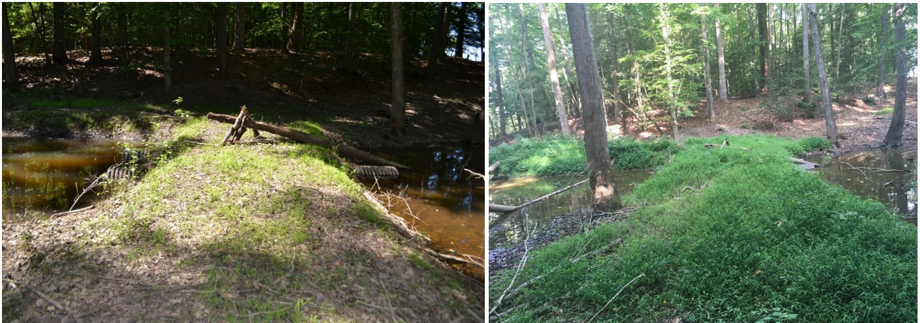
Figure 7: Second dam in the woods, photographed by Timothy Layton, Rapid Assessment Team, April 2017 on the left and Marian Norris 9/22/2017 on the right. Dam dimensions are 24 feet wide by 2.3 feet tall and the sediment level is halfway up the pipes. In September the vegetation is functionally emergent wetland.
