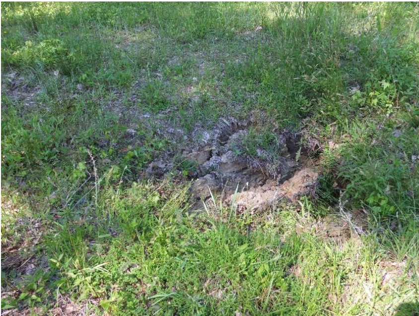
Figure 4: Sinkhole during Rapid Assessment Team visit in April 2017.
