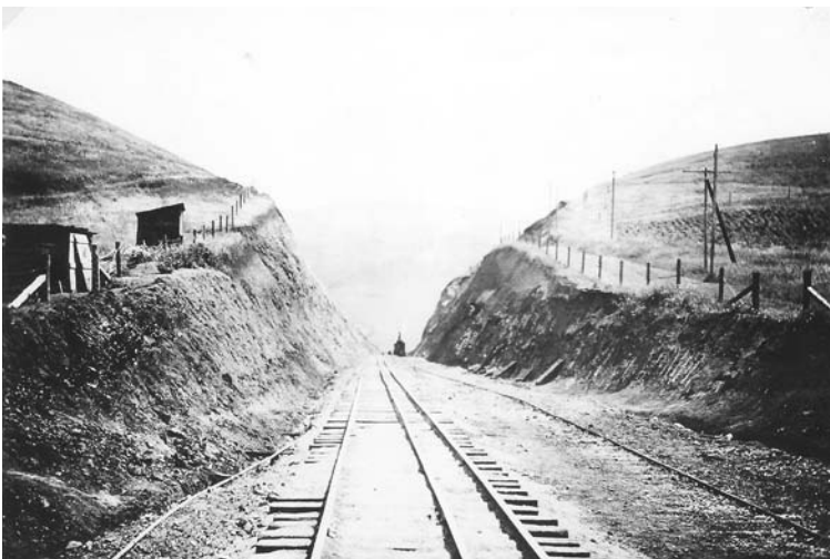
Fig. 4.3: Photo of the railroad cut south of Sharp Park (looking south).
