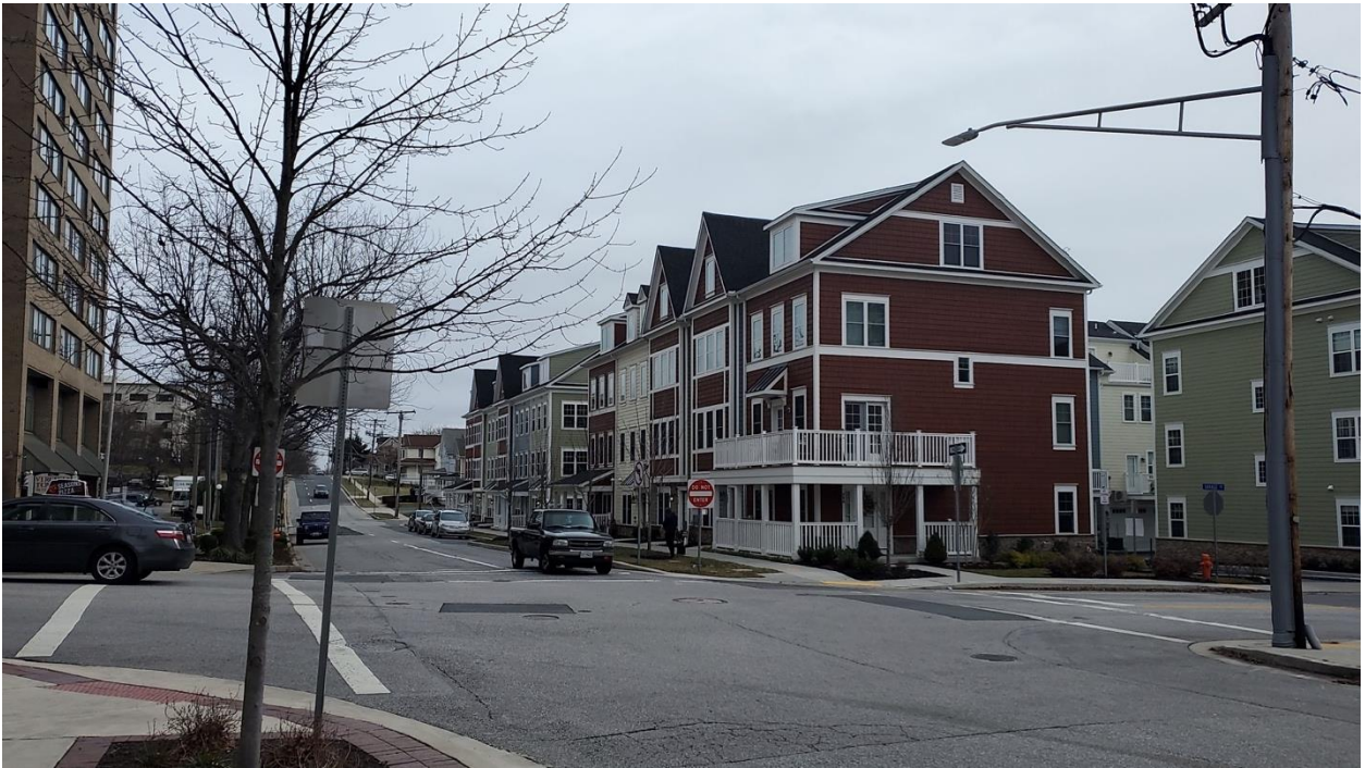
Figure 5.10 Towson Mews project at the entrance to East Towson
