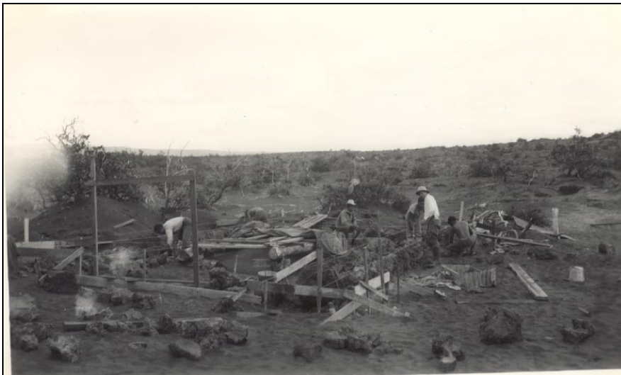
Construction of the Footprints shelter by the CCC. Photo courtesy of Hawai'i Volcanoes National Park.
