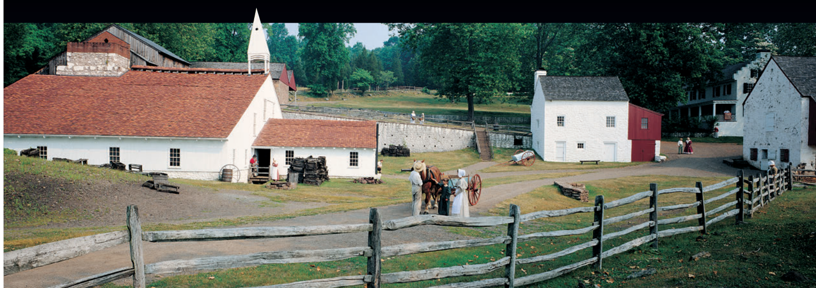
Molten iron was cast into stove plates and other products in the cast house, roofed with tiles to prevent fire
