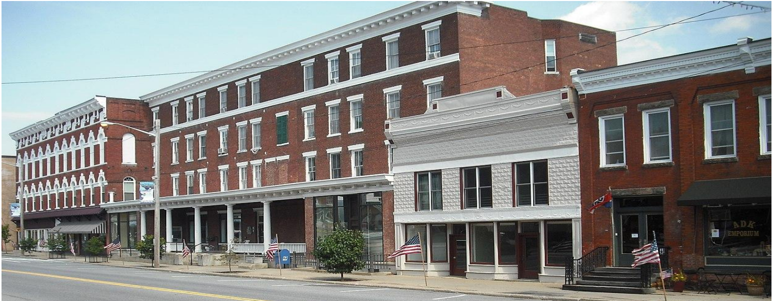
Essex County, NY - Town of Moriah, Hamlet of Port Henry. Main Street, Van Ornam & Murdock Block. Credit: Alex Scrodi
