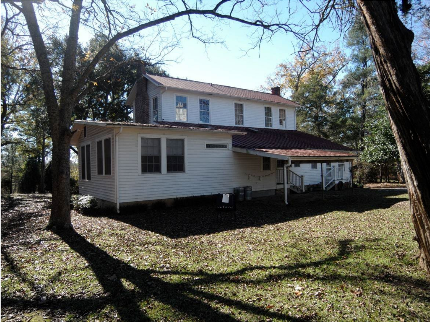
ANDALUSIA FARM (Flannery O'Connor Home) Milledgeville, Baldwin County, Georgia Main house, north (rear) and east facades showing 1959 addition Photograph by Evelyn Causey, November 2015
