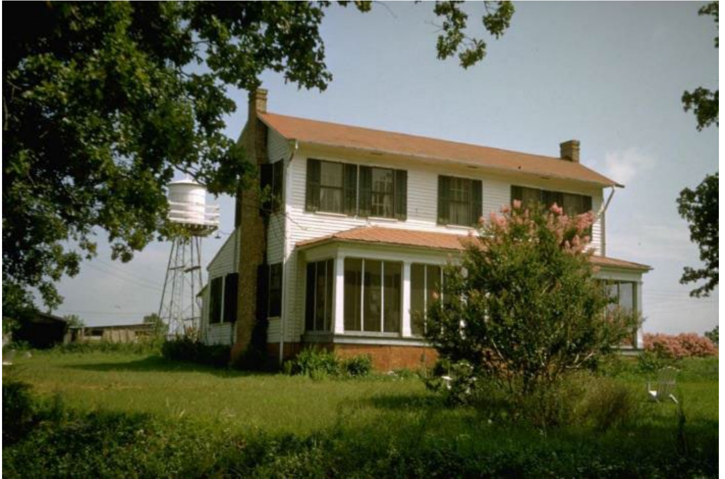
ANDALUSIA FARM (Flannery O'Connor House) Milledgeville, Baldwin County, Georgia Main house, 1950
