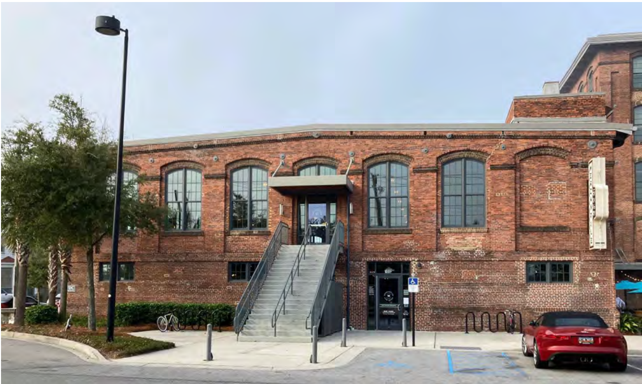
Photo 5: Former Picker House, east facade. Photograph by Rachel Donaldson, 2021.
