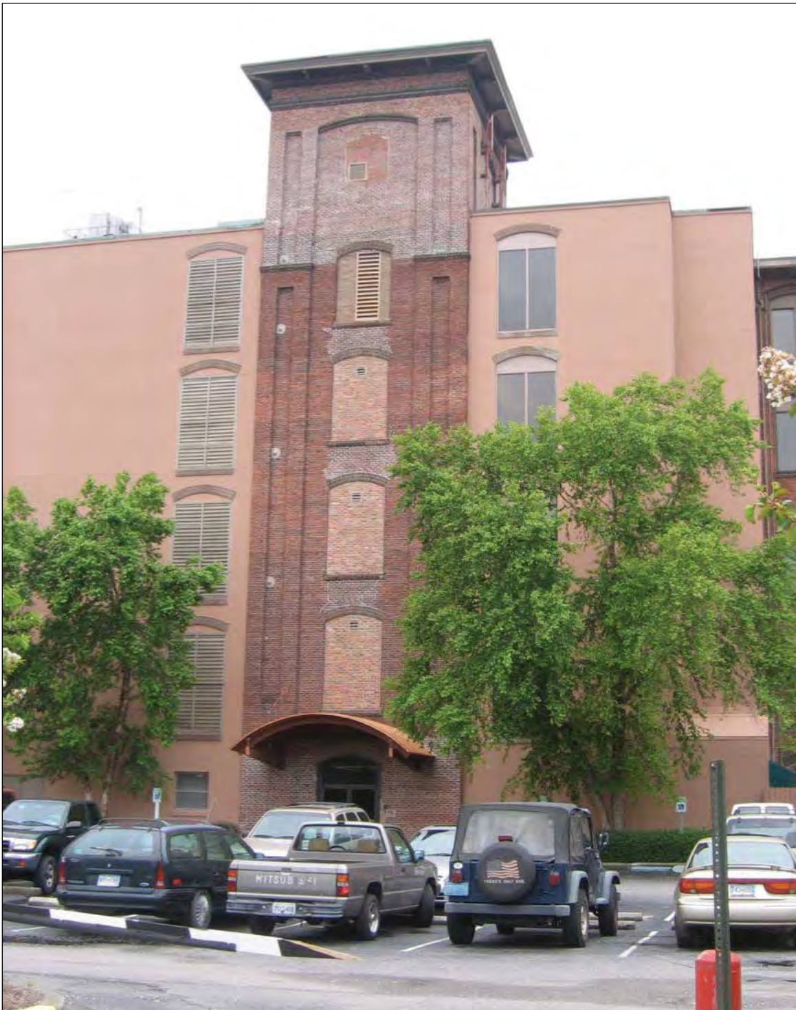
Figure 9. Main Mill, central tower, 2007. Image courtesy of Wecco Development, LLC.
