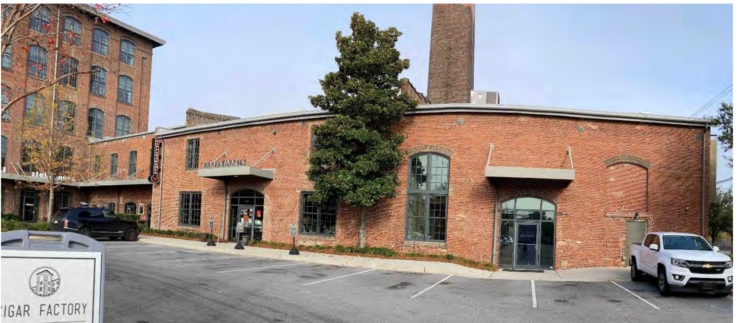
Photo 15: Boiler Room and Engine Room, south facade. Photograph by Rachel Donaldson, 2021.
