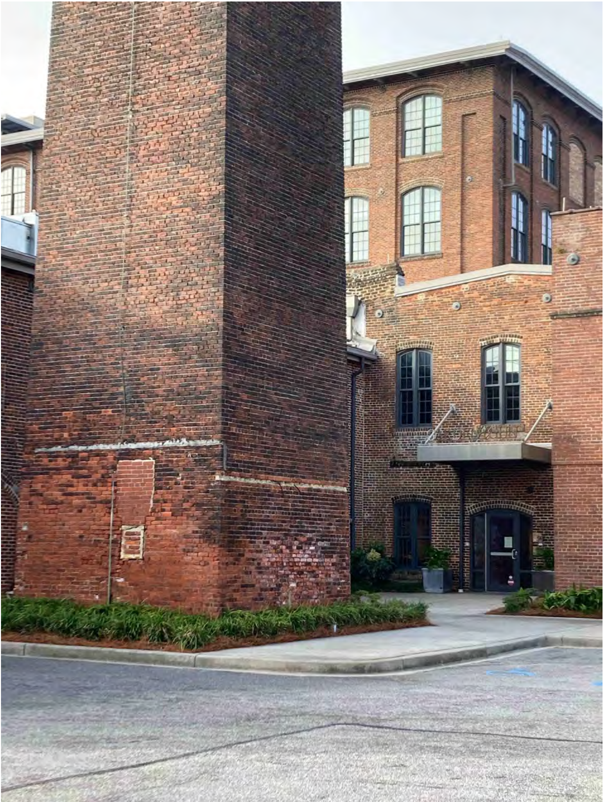
Photo 13: North Engine Room, east facade. Photograph by Rachel Donaldson, 2021.
