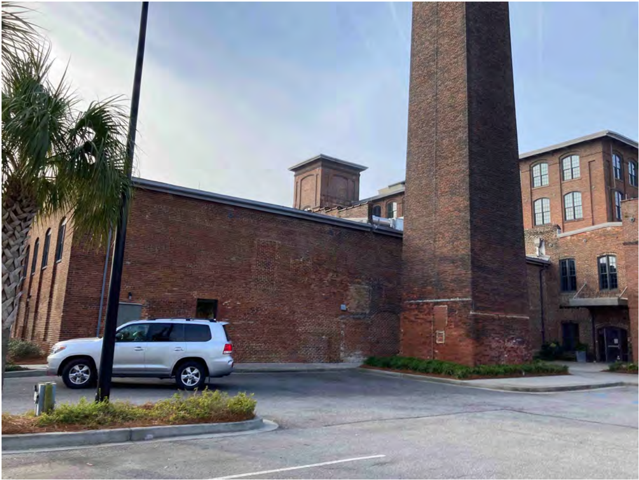
Photo 14: Smokestack and Boiler Room, north facade. Photograph by Rachel Donaldson, 2021.
