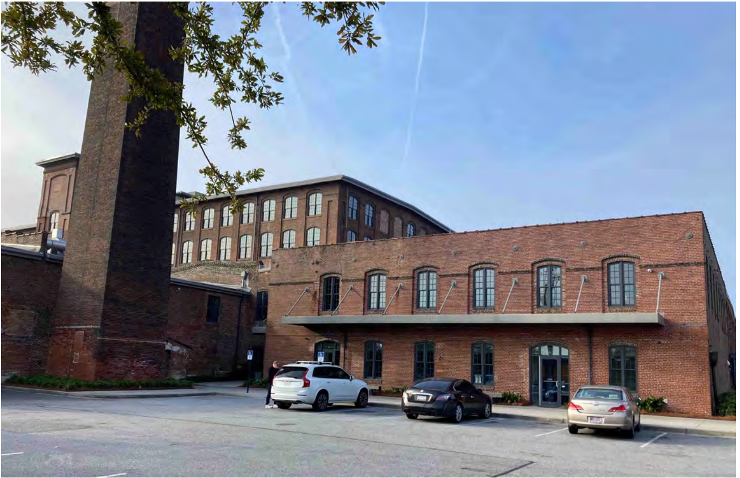
Photo 12: Building 8, east façade, and smokestack. Photograph by Rachel Donaldson, 2021.
