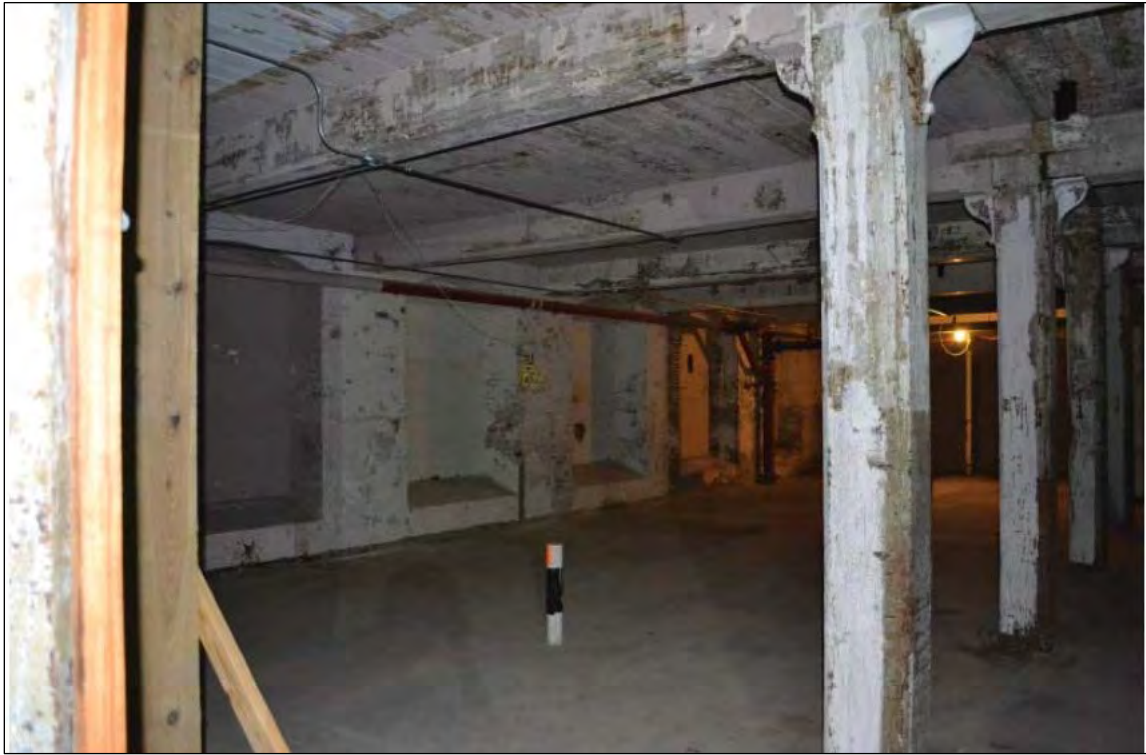
Photo 18: First floor, North Addition, looking south. Photograph by Wecco Development, LLC, 2013.
