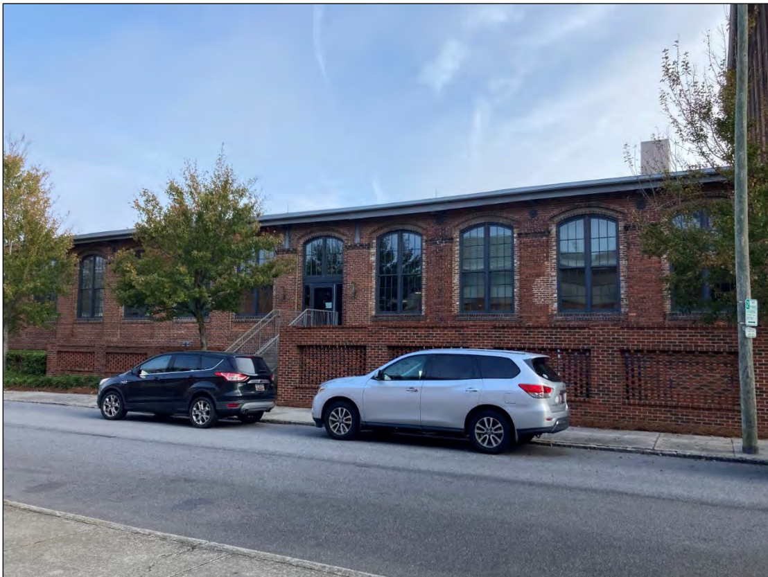
Photo 17: North Addition, west facade. Photograph by Rachel Donaldson, 2021.
