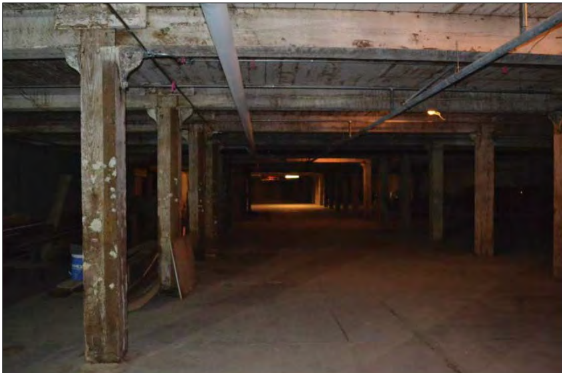
Photo 21: First floor, Main Mill, looking south. Note the chamfered post corners and absence of a ceiling, both elements of slow-burn mill construction. Photograph by Wecco Development, LLC, 2013.
