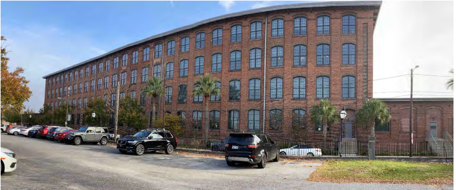
Photo 10: Main Factory and Office, west facade. Photograph by Rachel Donaldson, 2021.
