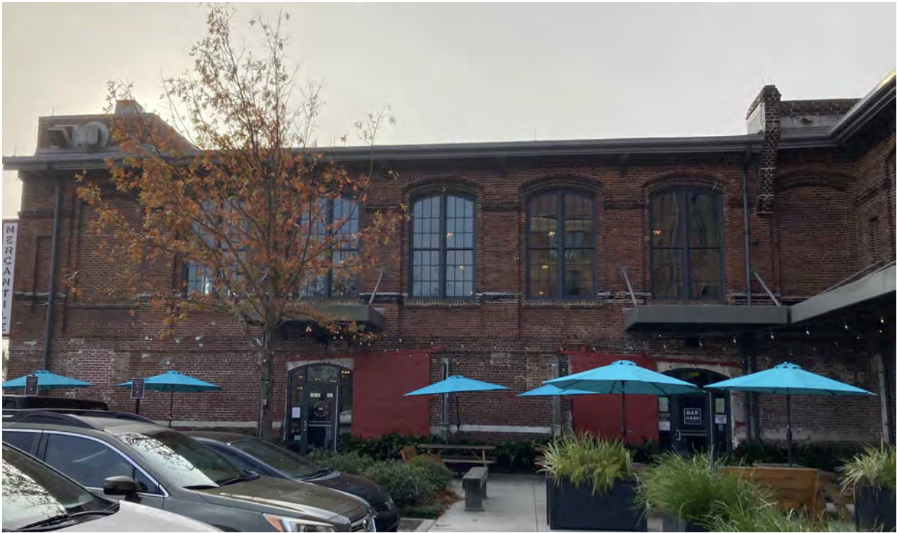
Photo 4: Former Picker House, north facade. Photograph by Rachel Donaldson, 2021.
