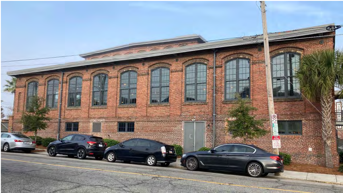
Photo 6: Former Picker House, south facade. Photograph by Rachel Donaldson, 2021.
