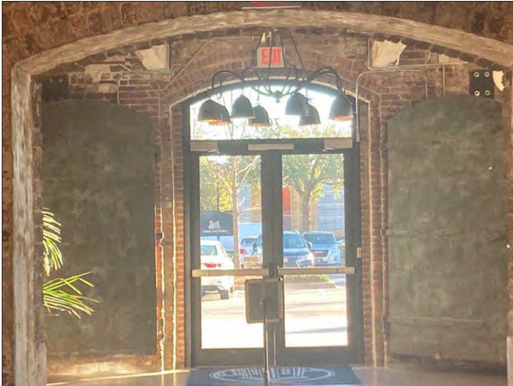
Photo 26: Entryway, first floor, Main Mill. Photograph by Rachel Donaldson, 2022.
