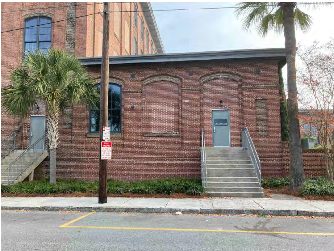
Photo 9: Office Building, west facade. Photograph by Rachel Donaldson, 2021.
