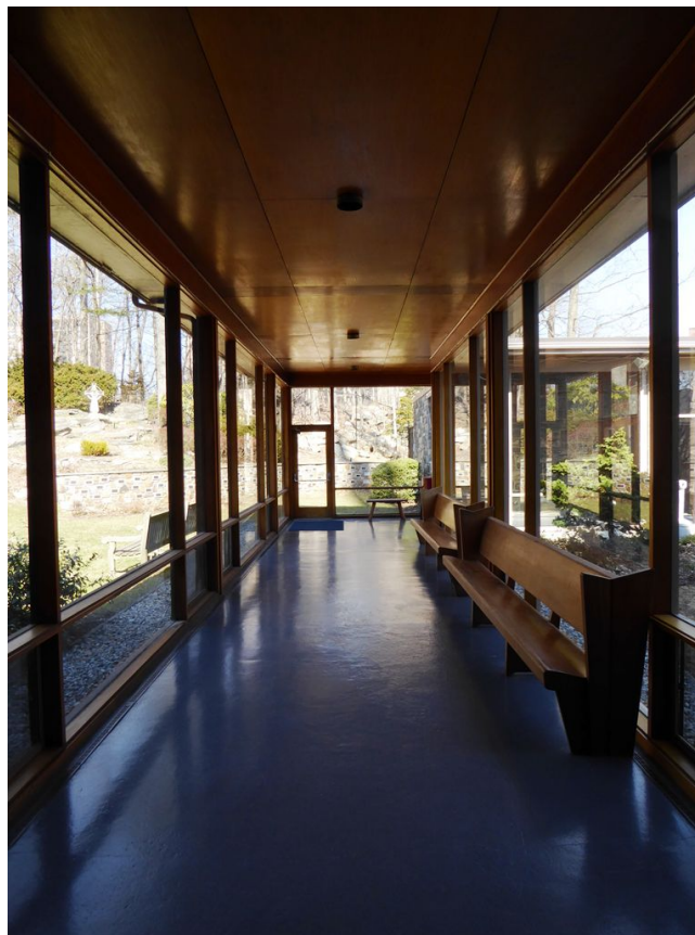
Figure 19: Parish unit, interior of hyphen passage, camera facing N from sanctuary narthex Photographer Wes Haynes, 2016
