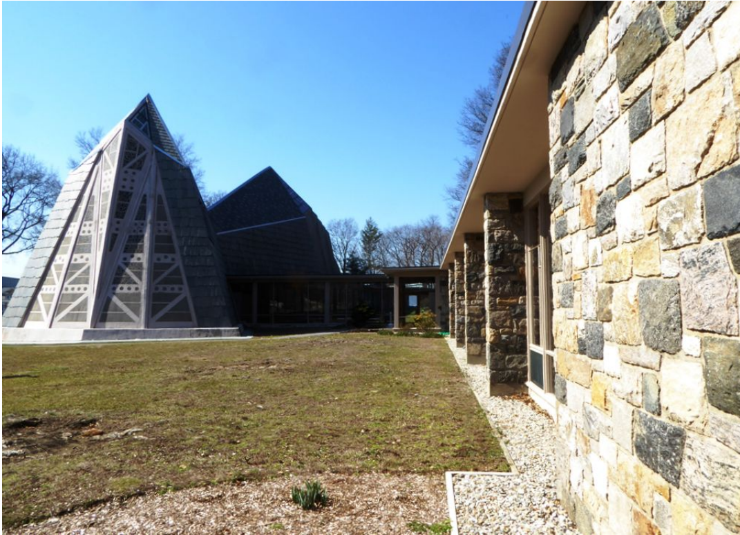
Figure 15: Sanctuary, East elevations; parish unit, south elevations of cloister wing and east elevation of hyphen passage, camera facing W within cloister Photographer Wes Haynes, 2016
