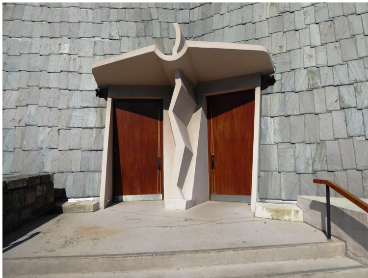
Figure 7: Sanctuary, south elevations, entrance portal, camera facing N Photographer Wes Haynes, 2016
