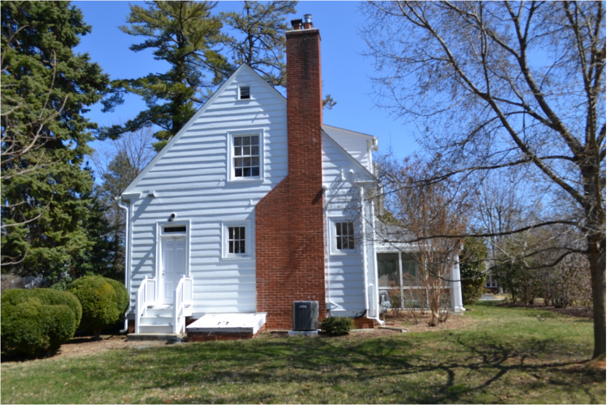
Photo 5. West side of cottage with entrance to the kitchen and the basement. The rear screen porch appears on the right.
