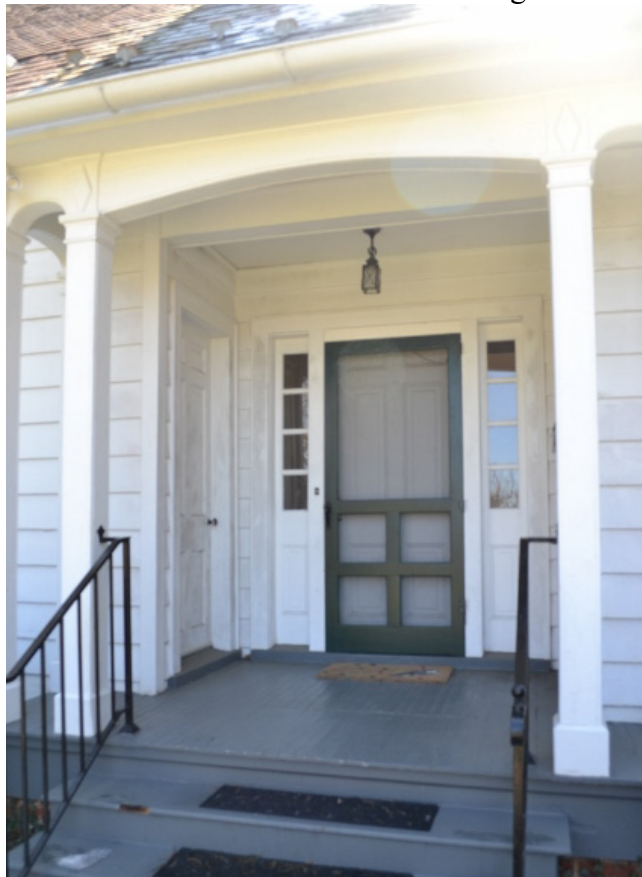
Photo 4. Close up view of front porch shows the primary door for visitors in the center and the secondary door for patients to the left.
