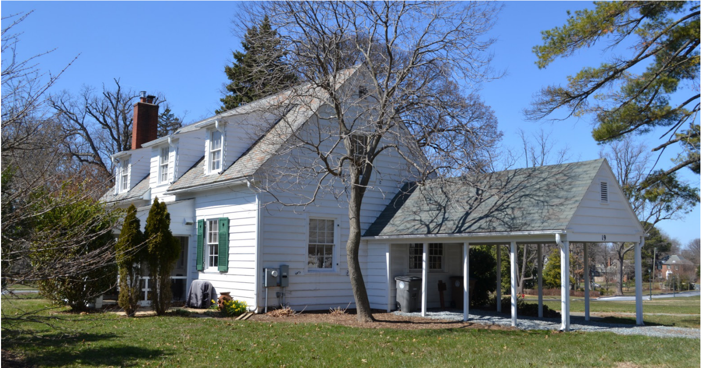
Photo 7. Rear and east side of cottage with carport.
