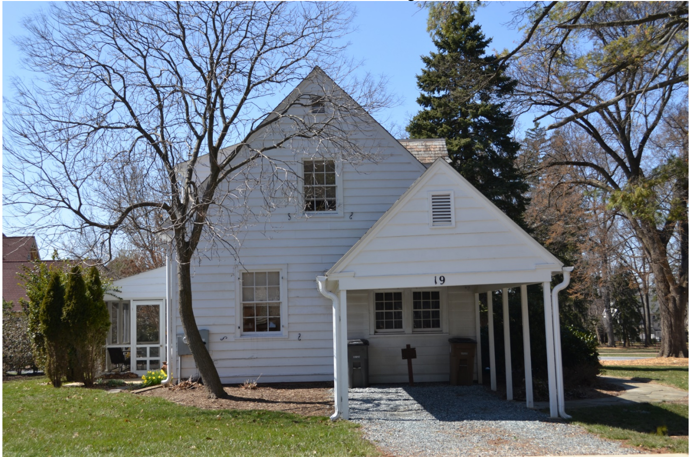
Photo 8. East side of cottage with carport. Windows on the wall below the carport appear to be the top half of a
