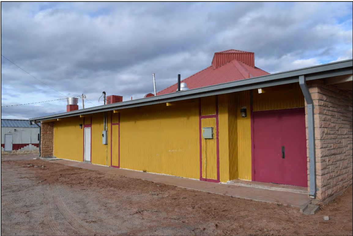
Photograph 4. Rear (southwest wall). View north.
