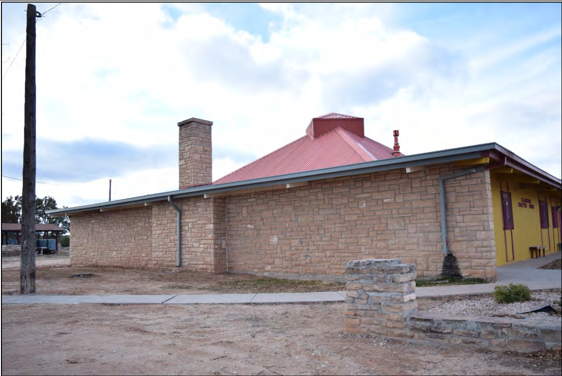
Photograph 3. Southeast wall with front to right. View west-northwest.
