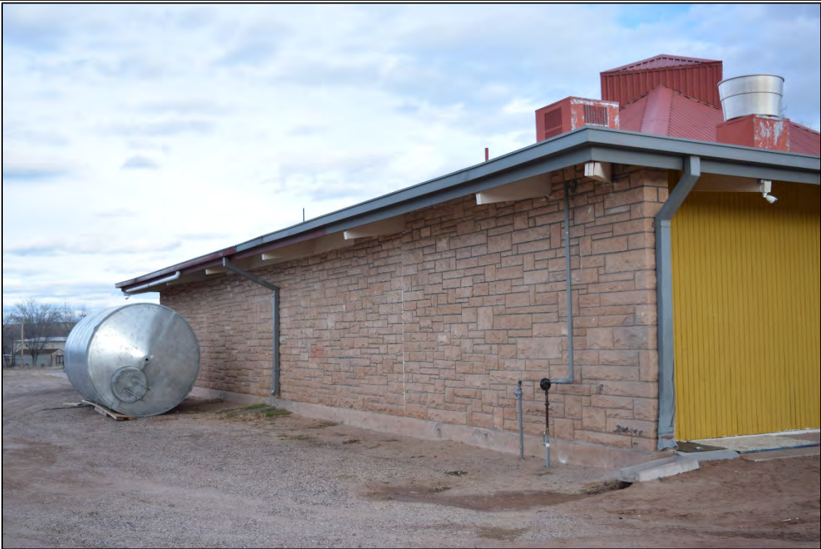
Photograph 5. Northwest wall with rear to right. View east.
