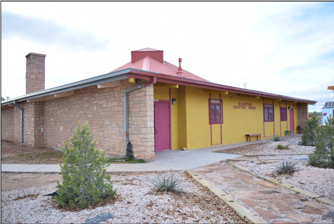
Photograph 1. Front and southeast walls. View west.
