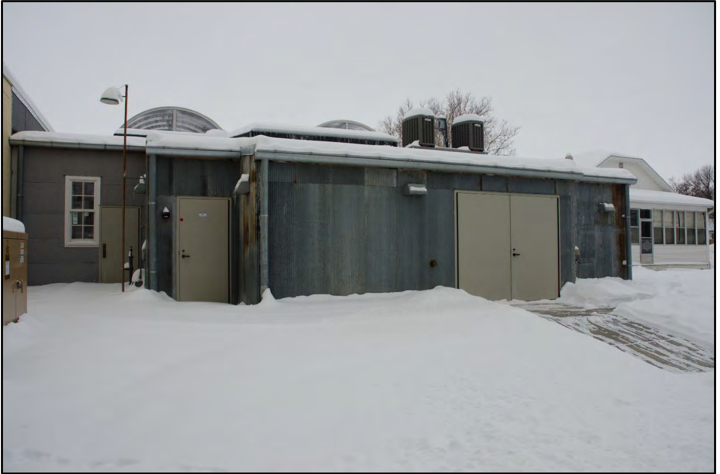
Photograph 5: KREGEL WINDMILL COMPANY FACTORY Nebraska City, Nebraska Exterior, north side; view south Photo by David Calease, January 2021
