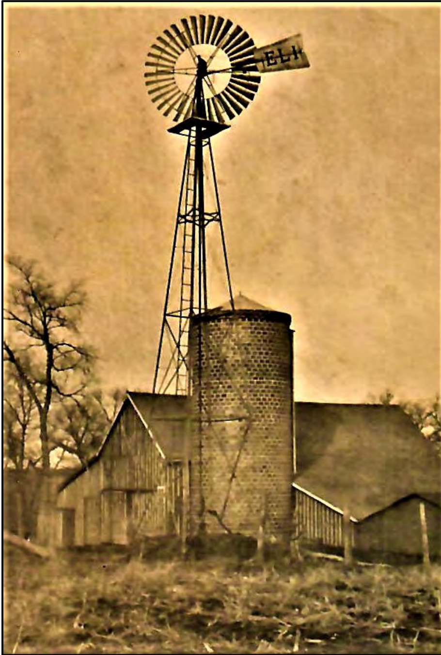
Figure 9: All steel ELI windmill on southeast Nebraska farmstead, ca. 1910. Courtesy of Kregel Windmill Factory Museum.
