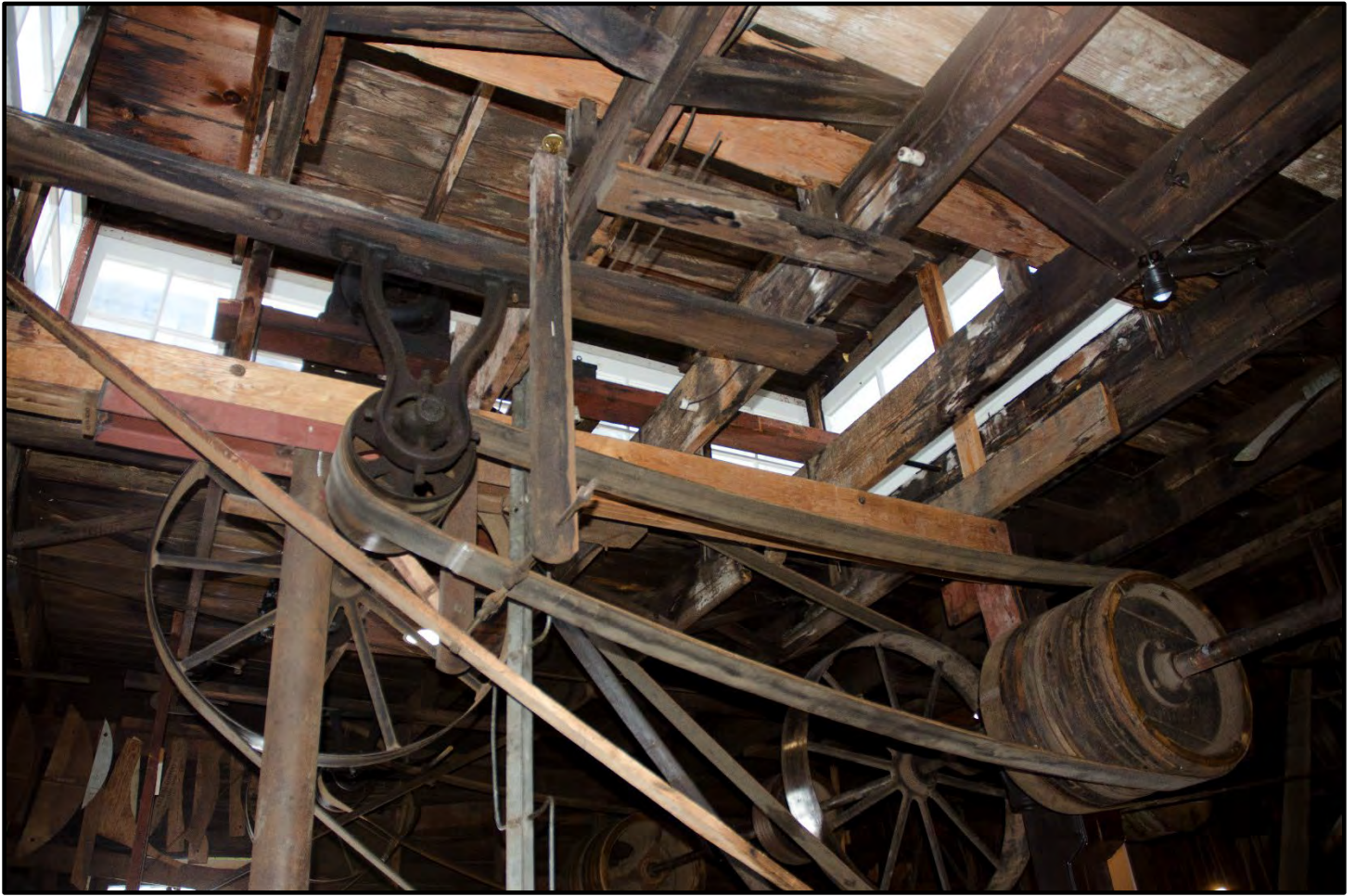
Photograph 14: KREGEL WINDMILL COMPANY FACTORY Nebraska City, Nebraska Interior, monitor and pulley-driven equipment Photo by David Calease, January 2021
