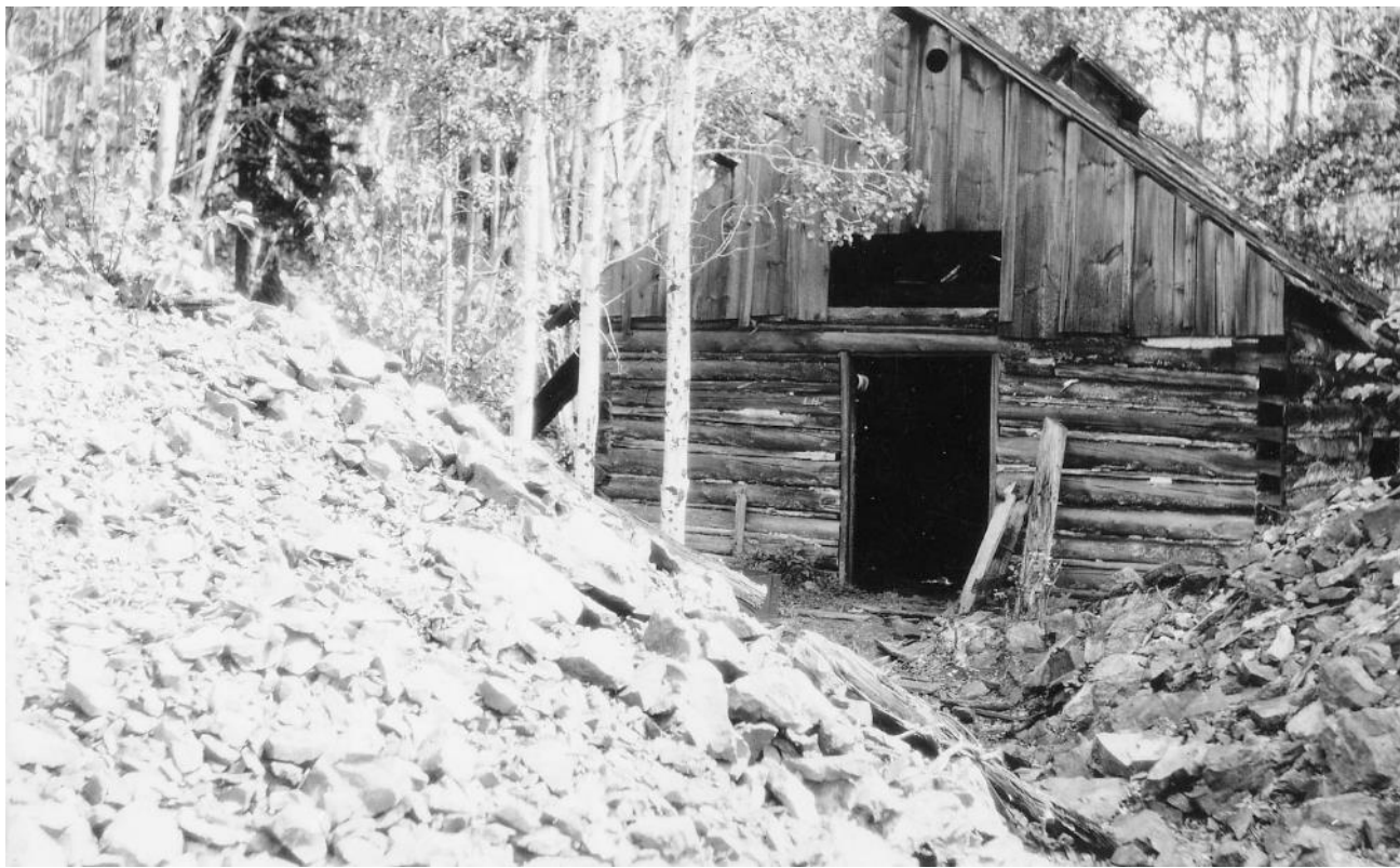
Figure 10: Ruins of Minong Mining Company blacksmith shop building ca. 1930s. View to the northeast. Fred Dustin Collection, Isle Royale National Park Archives.
