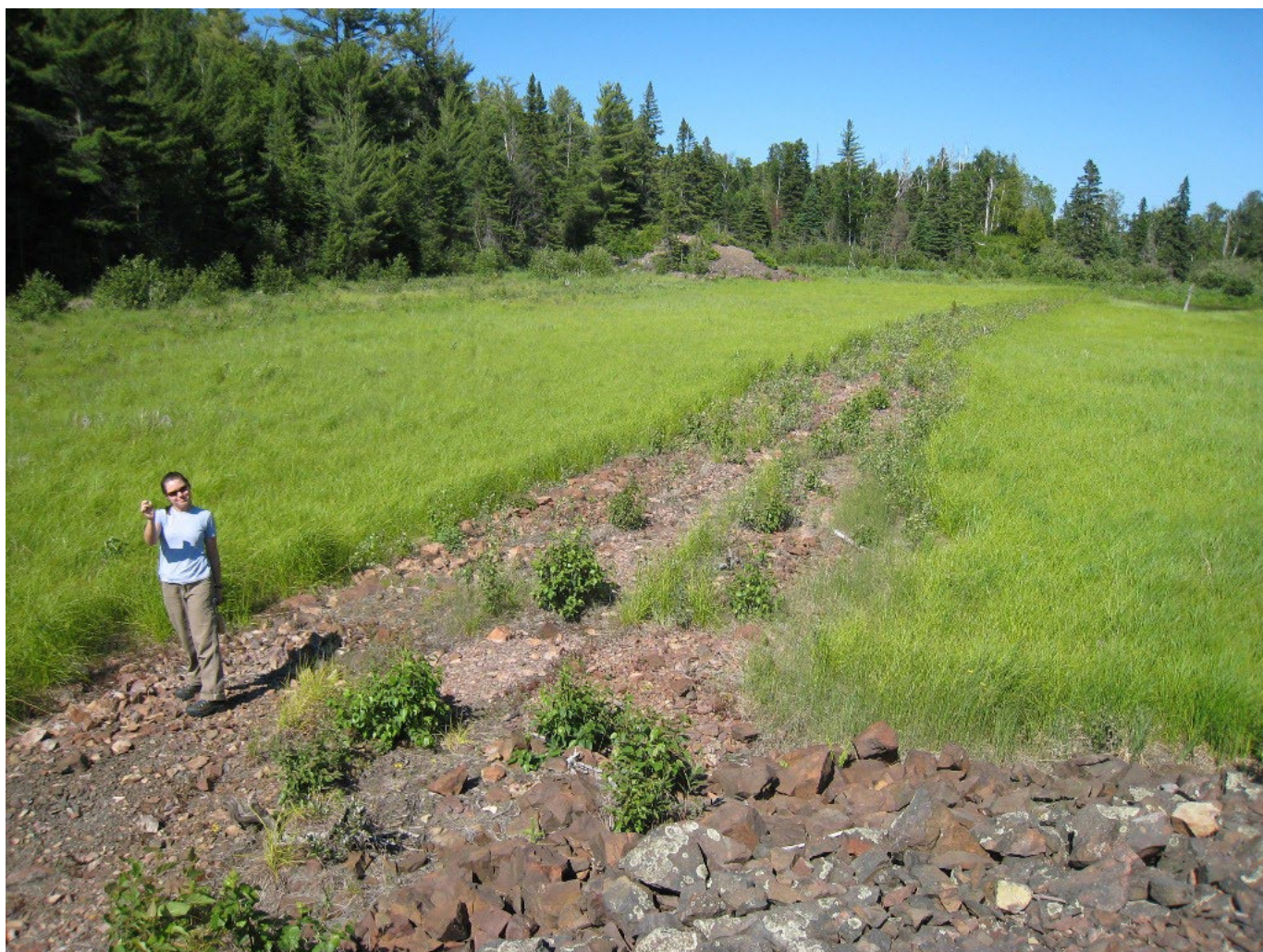
Figure 18: The Minong Mining Company Tramway remains as they appear today (2009). Photo facing northeast, towards McCargoe Cove. Seth DePasqual, Isle Royale National Park.
