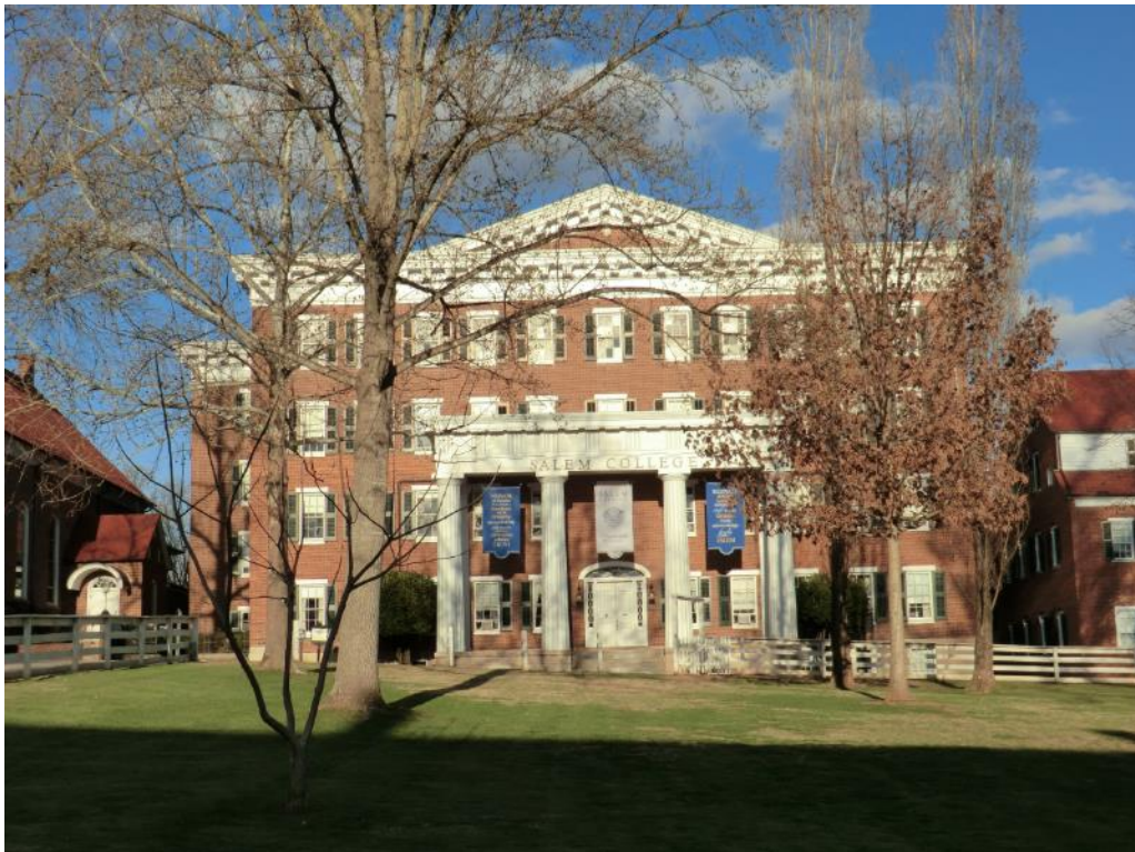
Main Hall, west façade. Martha B. Hartley Photographer, April, 2013
