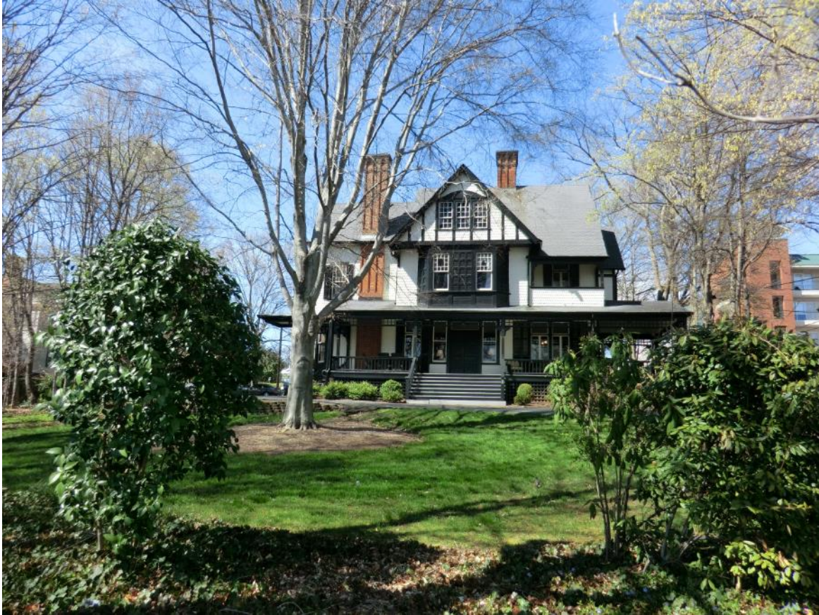
Hydehurst. South façade looking north. Martha B. Hartley Photographer, April, 2013
