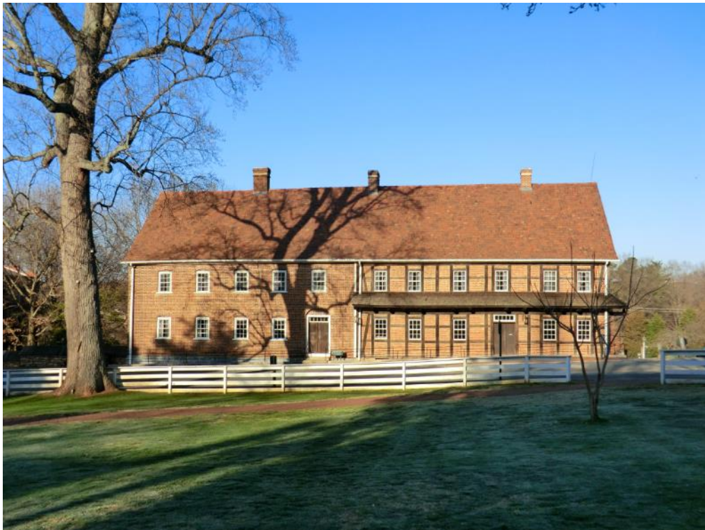
Single Brothers' House, east façade. Martha B. Hartley Photographer, April, 2013
