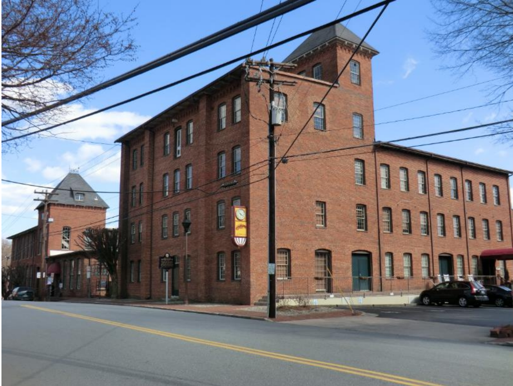
Arista Mill facing Brookstown Avenue, looking east. Martha B. Hartley Photographer, April, 2013
