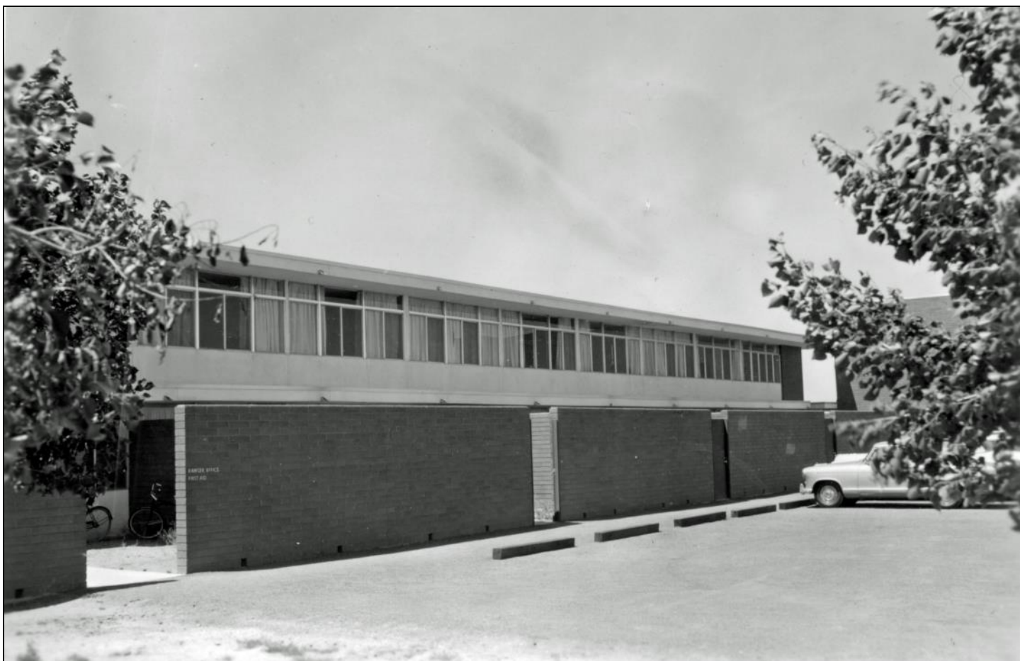
Figure 20. The front (east wall) of the apartment wing featured a band of windows on the second story and walled courtyards for the ground floor units. The community building is to the right in this ca. 1960s photograph. Courtesy Petrified Forest National Park, photographic archives, undated.
