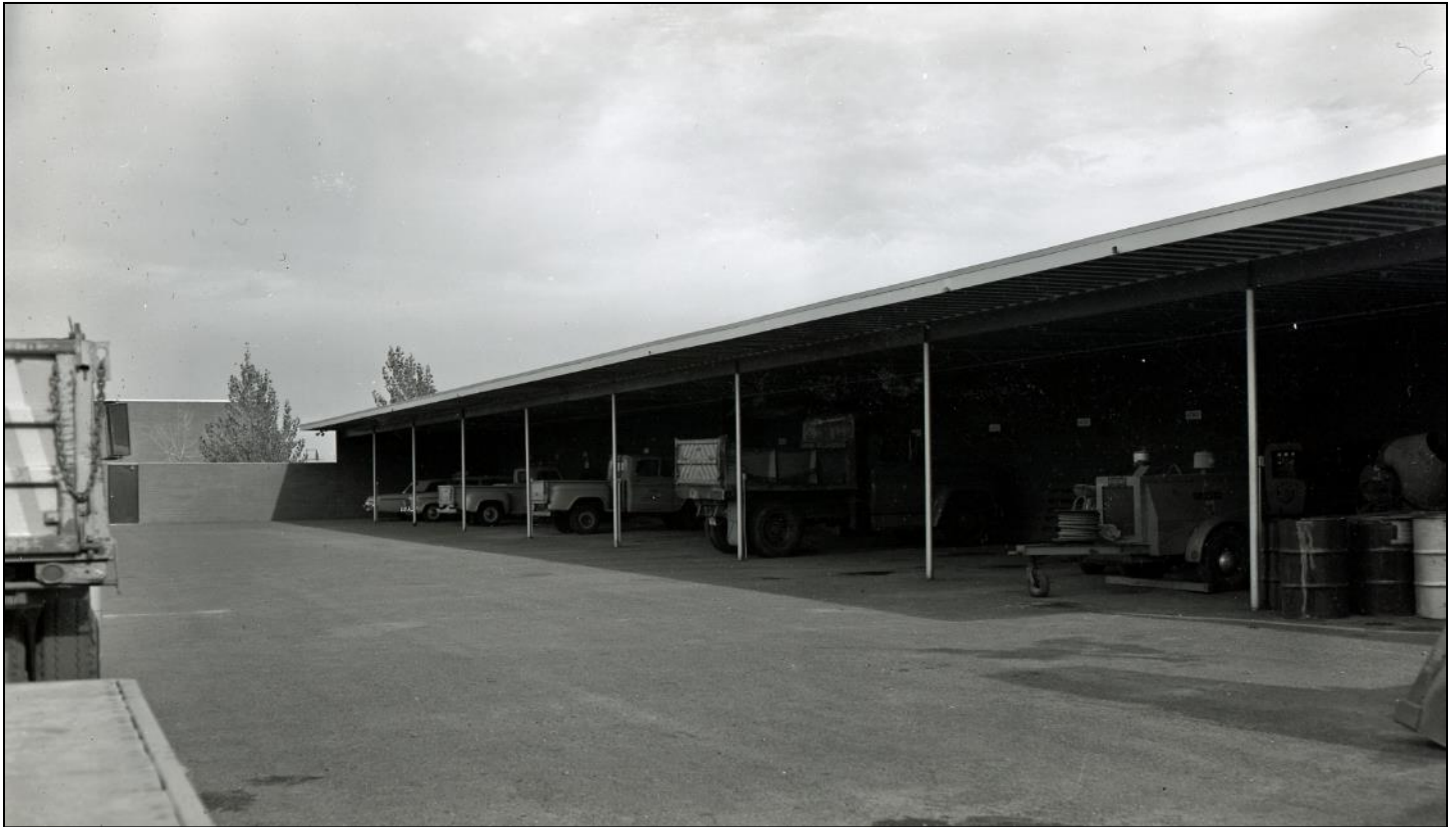
Figure 29. The vehicle storage building consisted of a series of open bays. This ca. 1960s view also shows the community building in the distance. Courtesy Petrified Forest National Park, photographic archives, undated.
