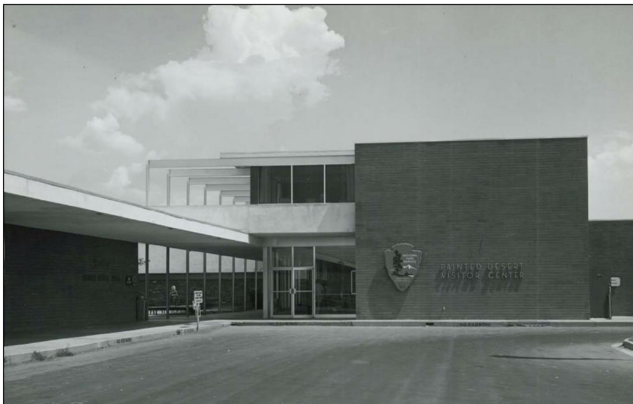
Figure 18. The visitor center/administration building is the focus of this 1963 photograph, with its glass curtain wall and second-story terrace with spider legs. The Painted Desert Oasis concession building is to the left. The apartment wing and plaza are visible in the opening between those two buildings. Courtesy Petrified Forest National Park, photographic archives, Philip Hyde, photographer, 1963.
