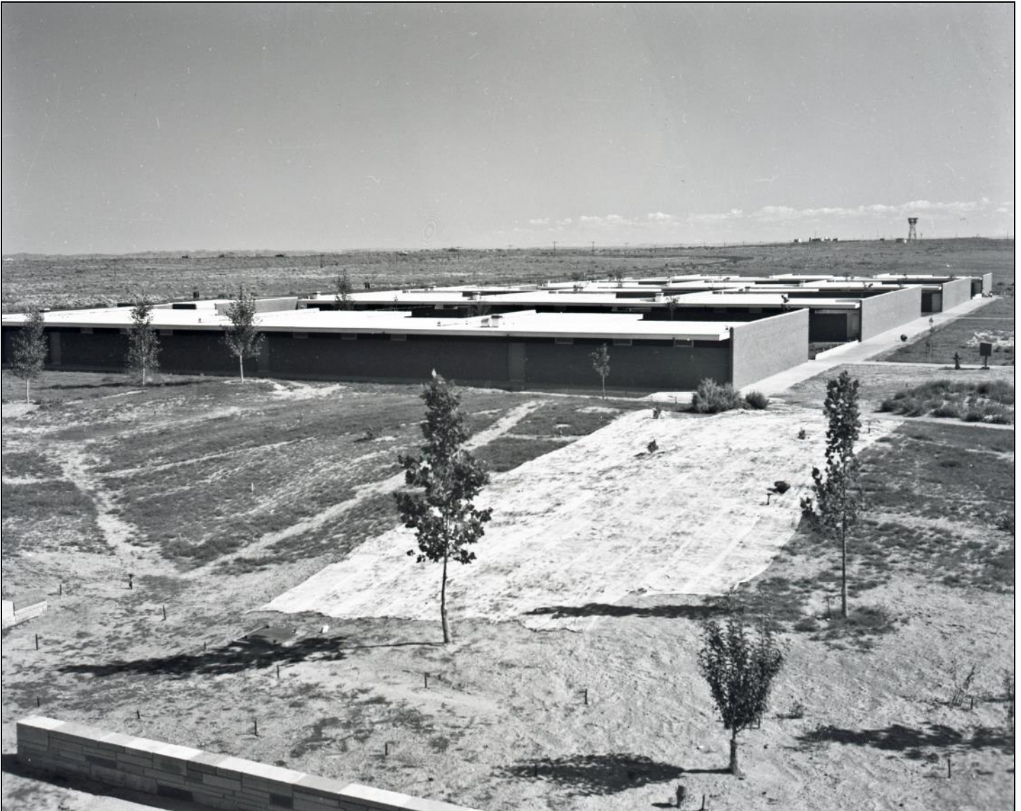
Figure 24. The four residence blocks are shown in this view from the roof of the apartment wing, ca. 1960s. Courtesy Petrified Forest National Park, photographic archives, undated.
