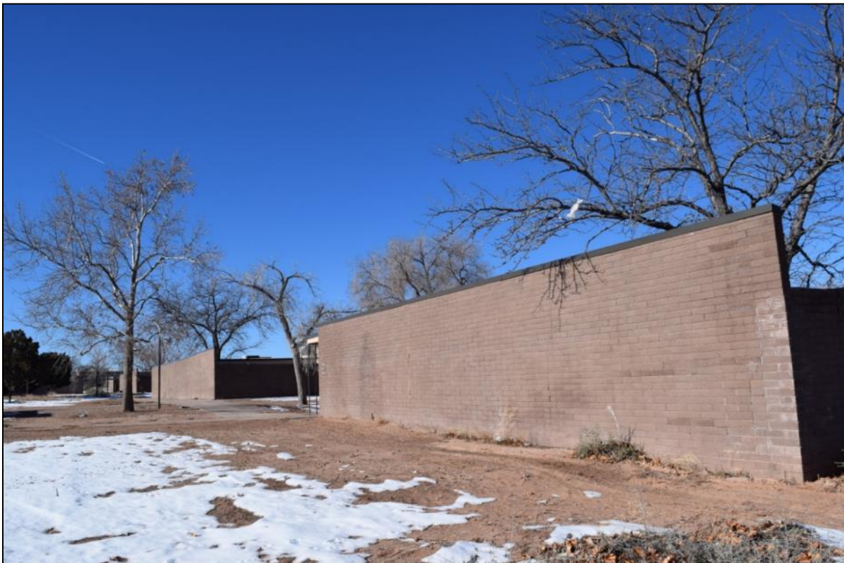
Photograph 24. Residence block showing east walls of blocks A through D (left to right, Resources 13, 14, 15, and 16).
