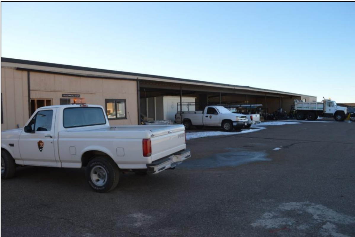
Photograph 38. Vehicle storage building (Resource 29), front (west wall).
