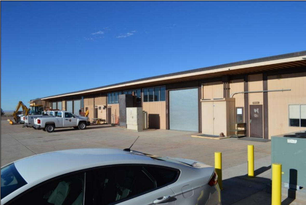
Photograph 37. Maintenance building (Resource 28), front (east wall).
