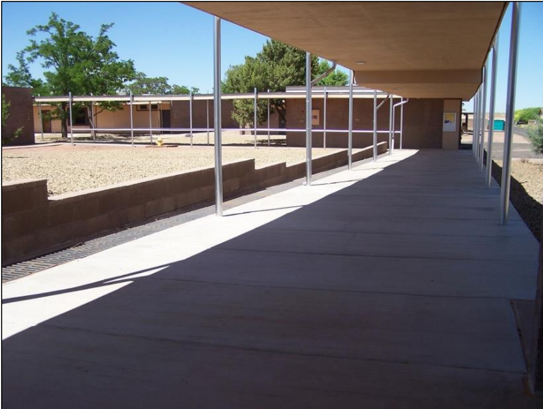
Photograph 17. Covered walkway (Resource 6), with residence blocks A and B to left (Resource 13 and 14, respectively) and carport (Resource 21) to right.
