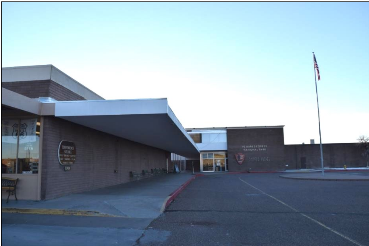
Photograph 2. Visitor center (Resource 1) in distance with Painted Desert Oasis concession building to left (Resource 2).
