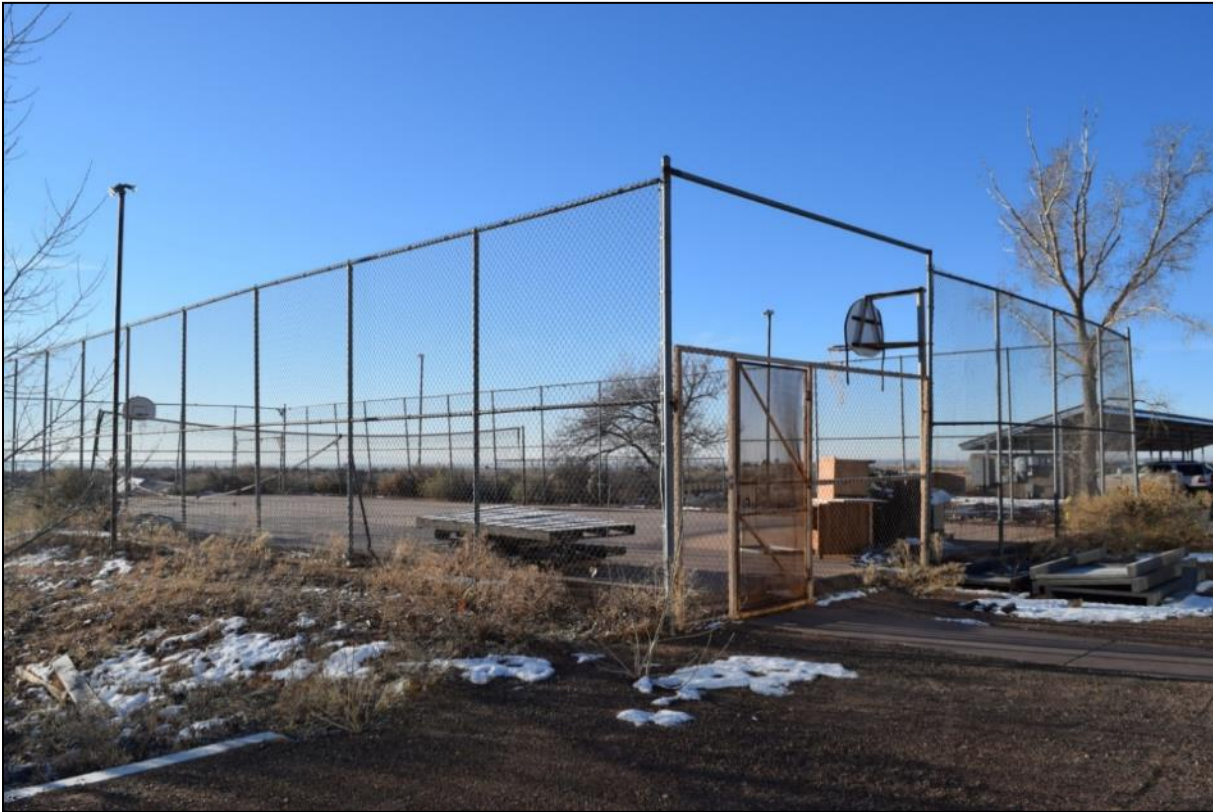
Photograph 23. Basketball/volleyball court (Resource 12) with the photovoltaic array (Resource 30) to the right.
