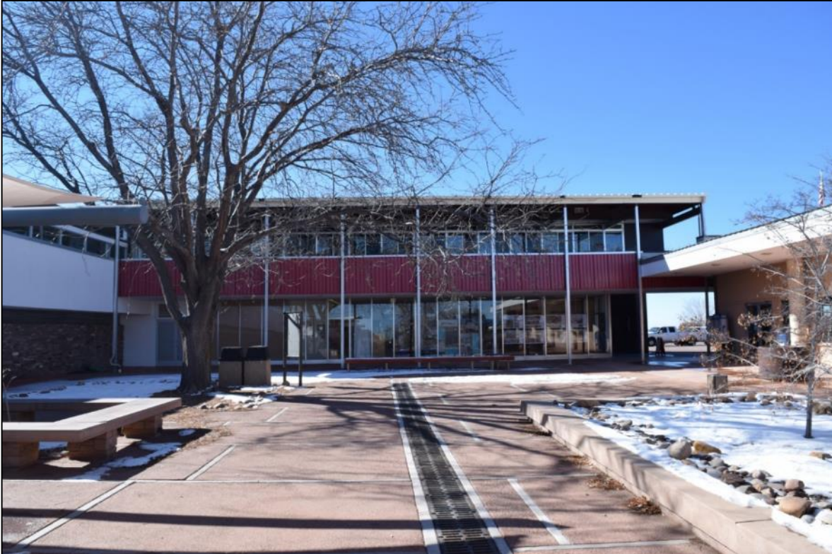
Photograph 13. Central plaza (Resource 4), with visitor center/administration building (center), Painted Desert Oasis (right), and apartment wing (left). Note sandstone bench to left.
