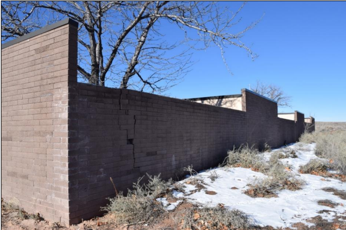
Photograph 29. Rear (north wall) of residence block D.
