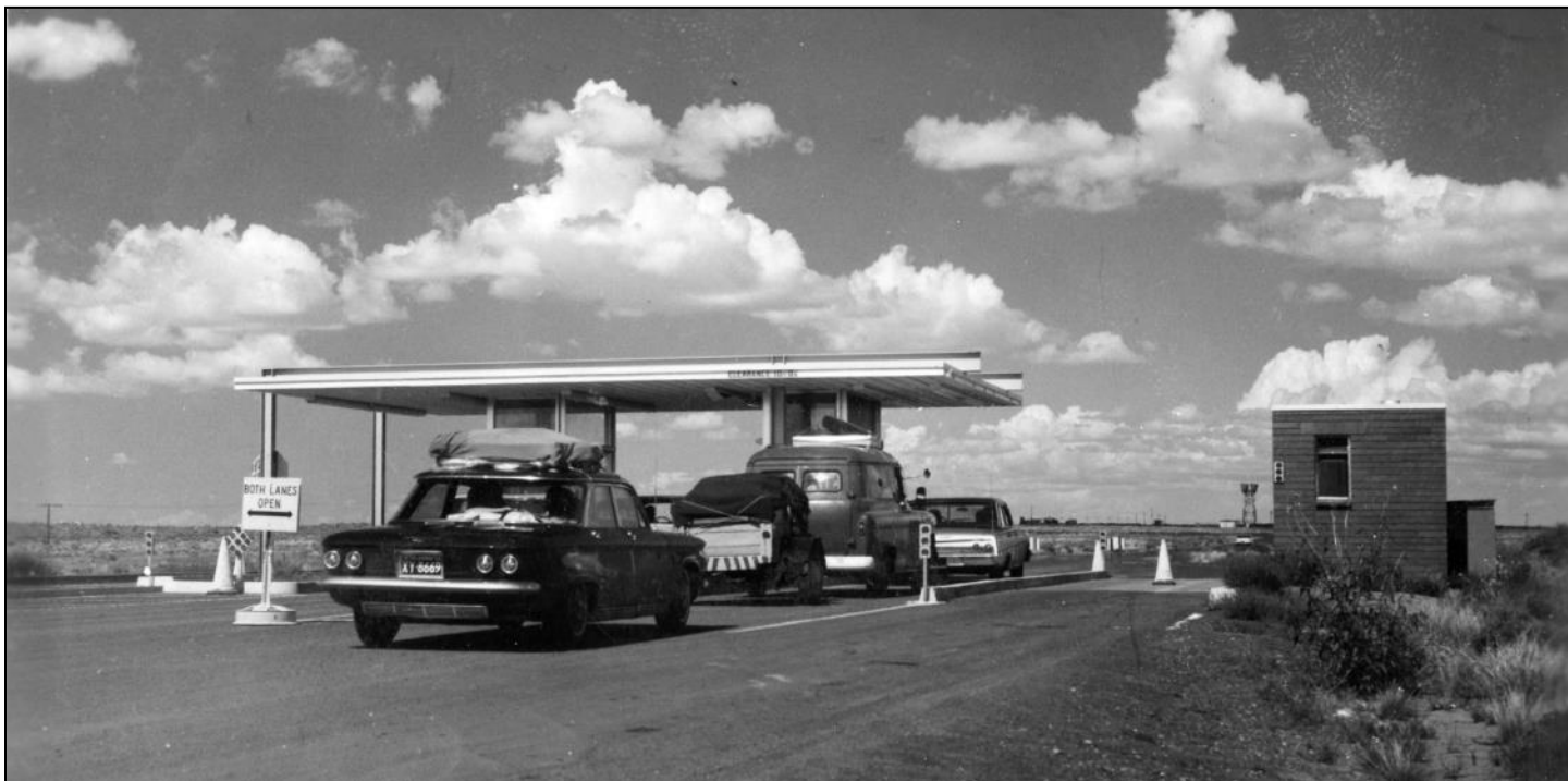
Figure 23. The entrance station in the middle of the road (no longer extant) is to the left and the entrance station at the edge of the road (right) are shown in this 1960s image. Courtesy Petrified Forest National Park, photographic archives, undated.
