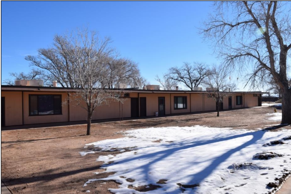
Photograph 27. Residence block C (Resource 15), front (south wall).
