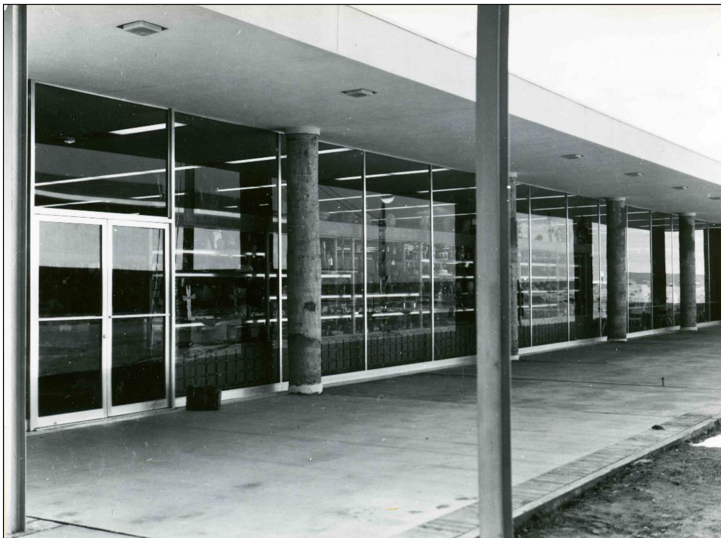
Figure 19. The Painted Desert Oasis concession building displays its glass curtain wall in this view; the narrow ceramic tiles have not yet been installed on the circular columns in front. Courtesy Petrified Forest National Park, photographic archives, ca. 1963-64.
