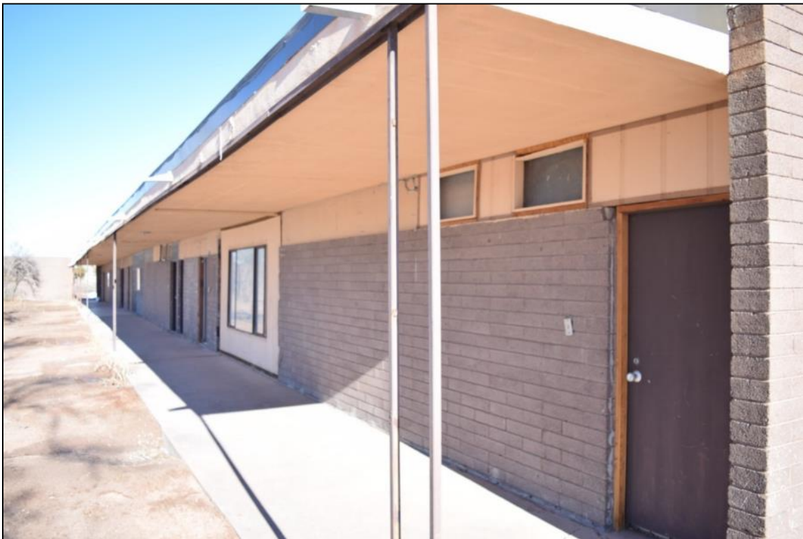
Photograph 28. Residence block D (Resource 16), front (south wall).
