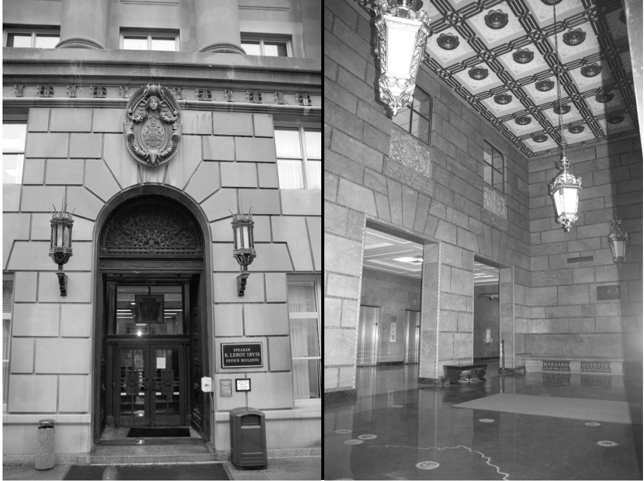
South Office Building, entrance detail (left)
