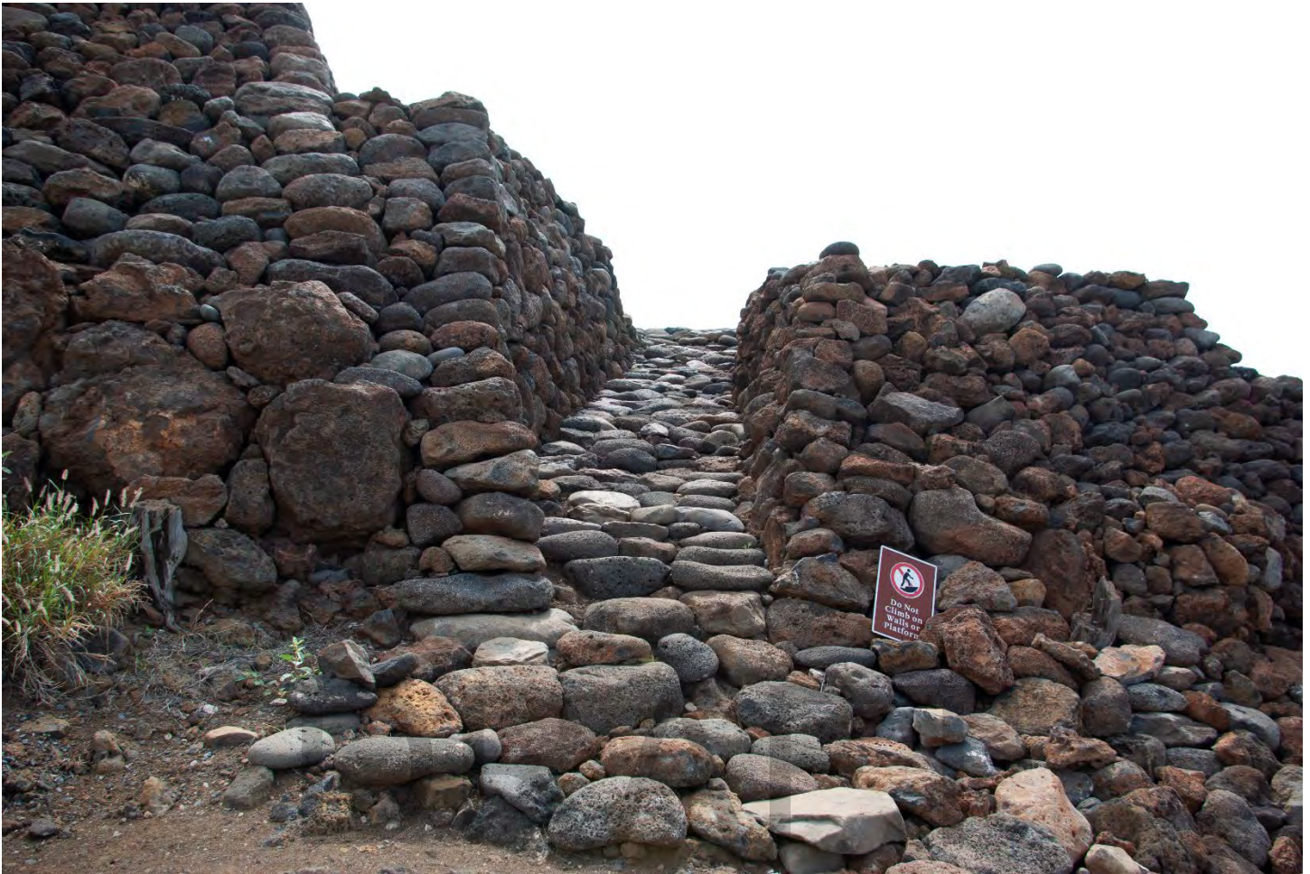
Photo #20 of 81 (HI_Hawaii_Puukohola Heiau NHL_0020) Pu'ukoholā Heiau, heiau entrance. Camera facing south.
