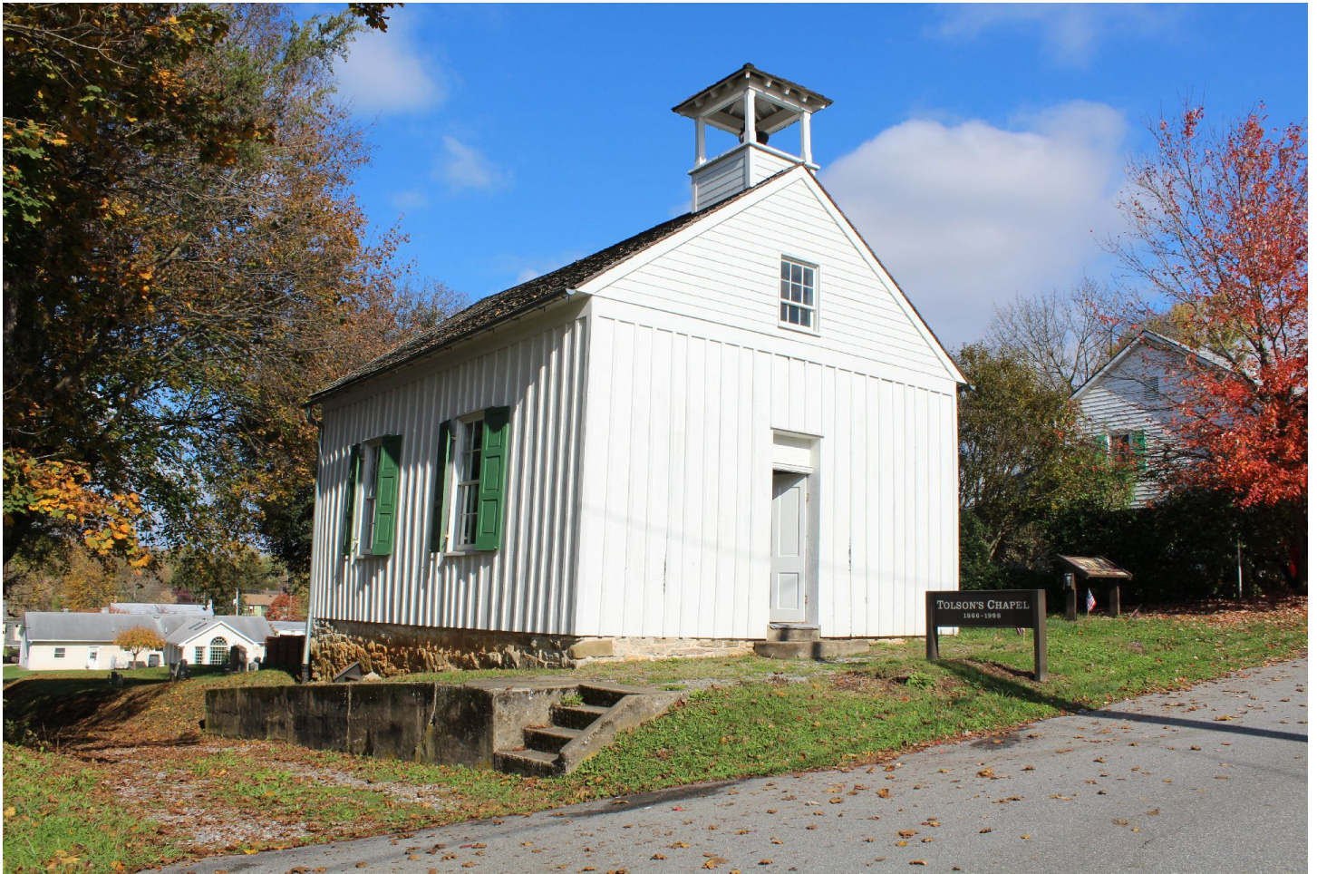
Photo 1 of 10. South and west elevations of church/school, looking northeast, showing west alley. November 2017.
