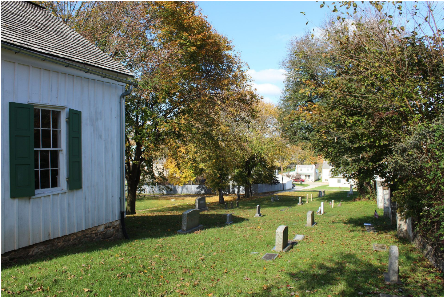
Photo 5 of 10. Cemetery, looking northwest from east property line, showing east elevation of church/school. November 2017.
