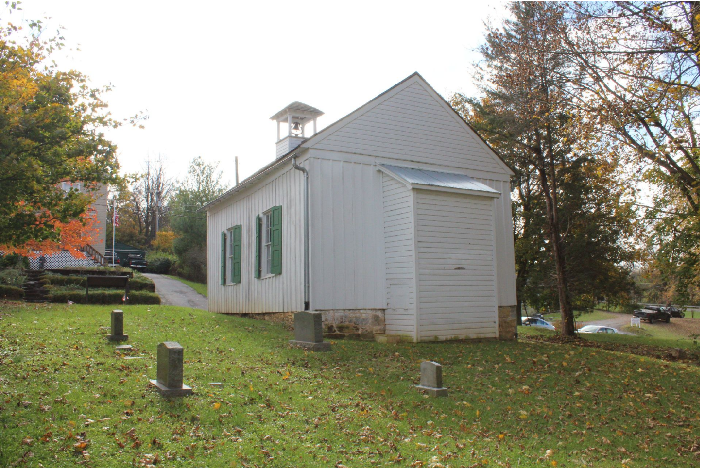
Photo 3 of 10. North and east elevations of church/school, looking southwest from cemetery towards East High Street with cemetery in foreground. November 2017.
