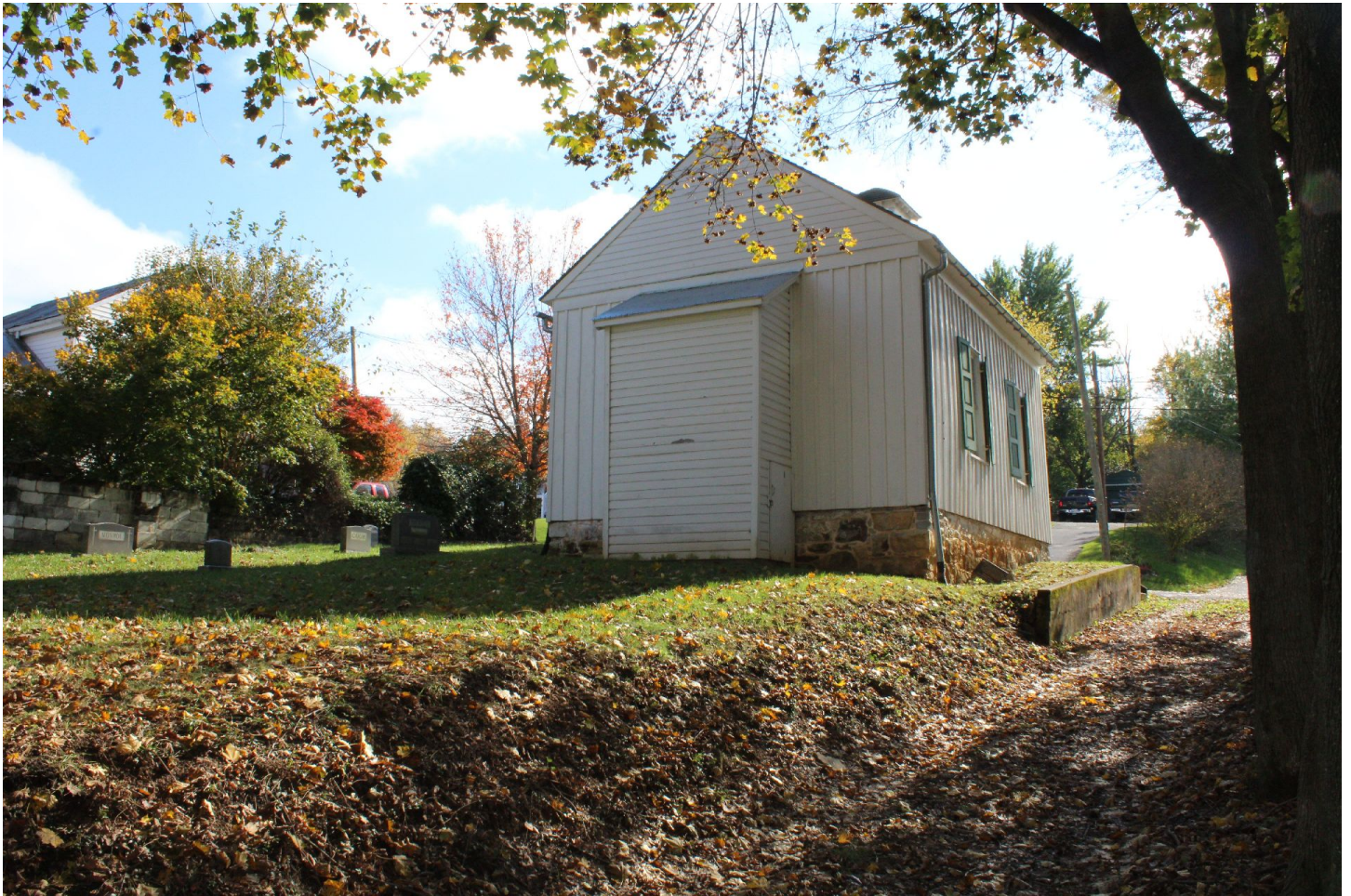
Photo 4 of 10. North and west elevations of church/school, looking southeast from west alley. November 2017.
