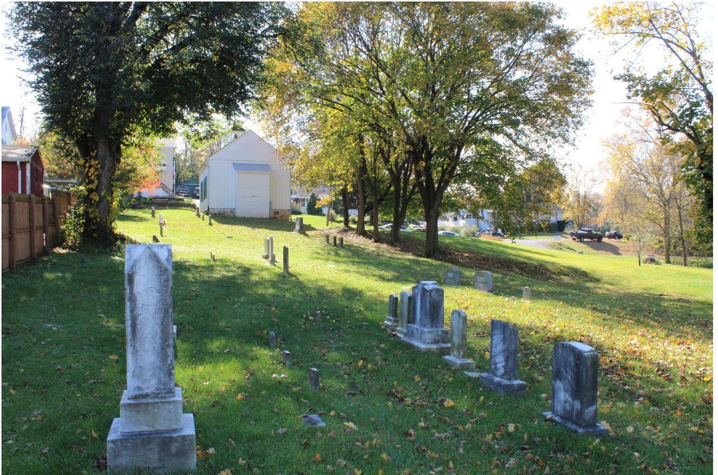
Photo 6 of 10. Cemetery, looking south from northeast corner of property, showing north elevation of church/school in background. November 2017.
