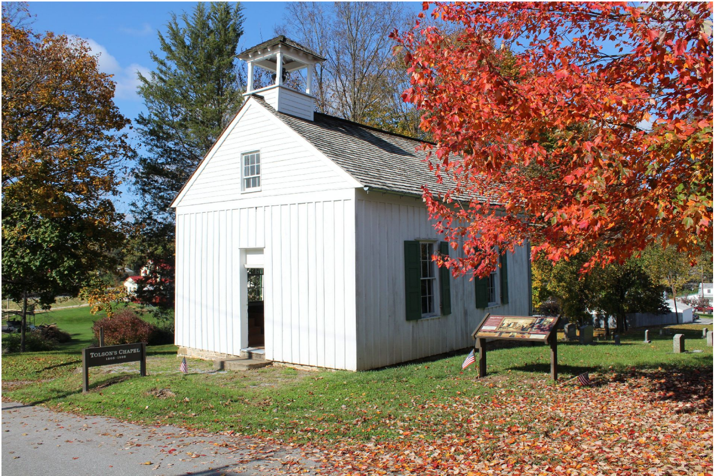
Photo 2 of 10. South and east elevations of church/school, looking northwest, showing southeast corner of cemetery. November 2017.
