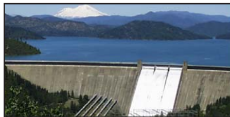
Shasta Dam, Shasta, California (Credit: BOR)
