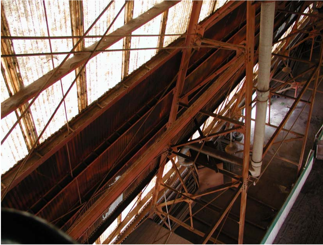
Vertical Truss and Diagonal Rod Bracing
