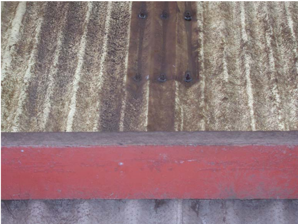
Vertical Splice at Translucent Sheathing
