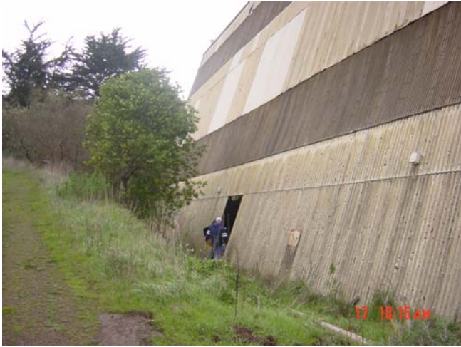
East Side Exterior
