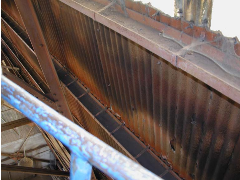
Wall Cladding Bracket Supports
