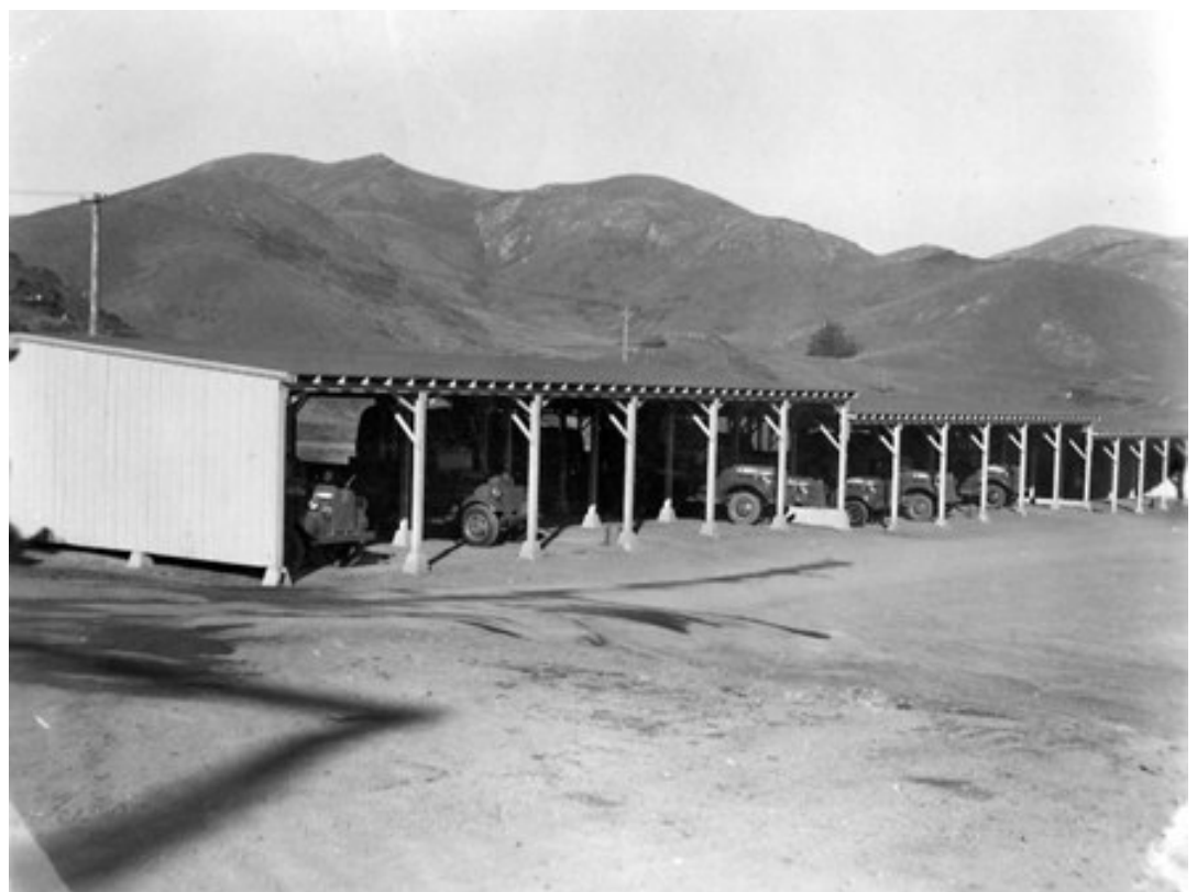
West Vehicle Shed, Ft Barry, 1942. (PARC, GOGA 32423)
