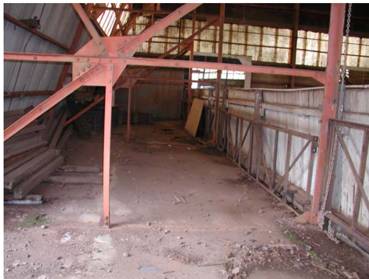
Vertical Truss facing South Wall
