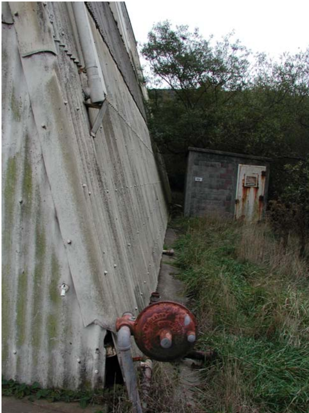
West Side Exterior
