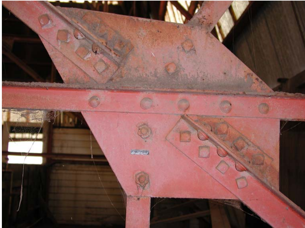
Splice Plate at Vertical Truss Field Bolts and Shop Rivets
