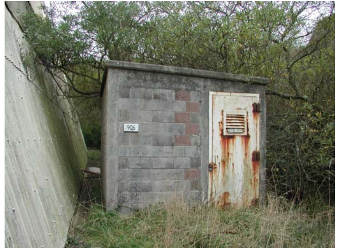
South Side Exterior
