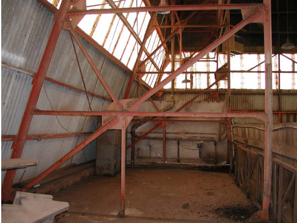
Vertical Trusses Facing North Wall
