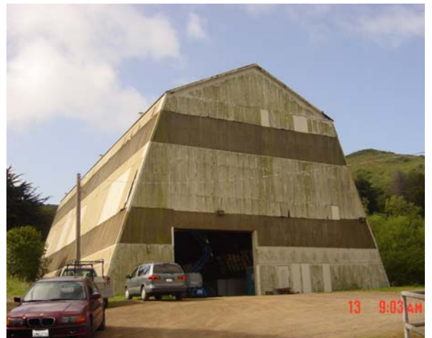
North Side Exterior
