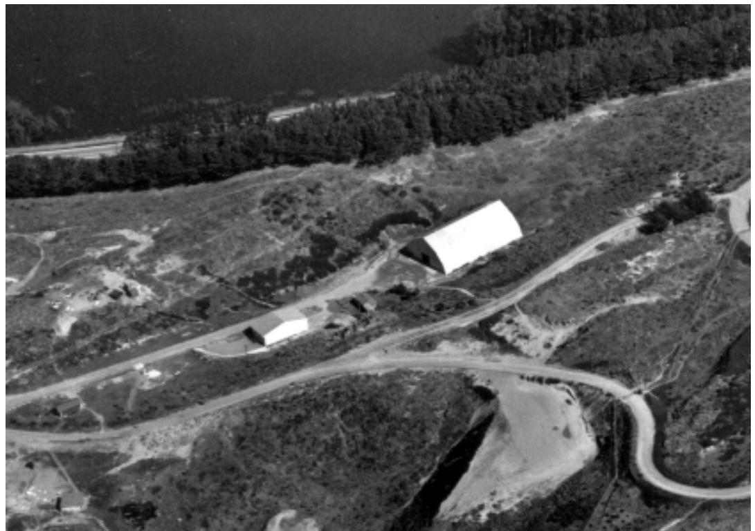
Ft. Funston Balloon Hangar, San Francisco, 1942 (now demolished). (PARC, GOGA)
