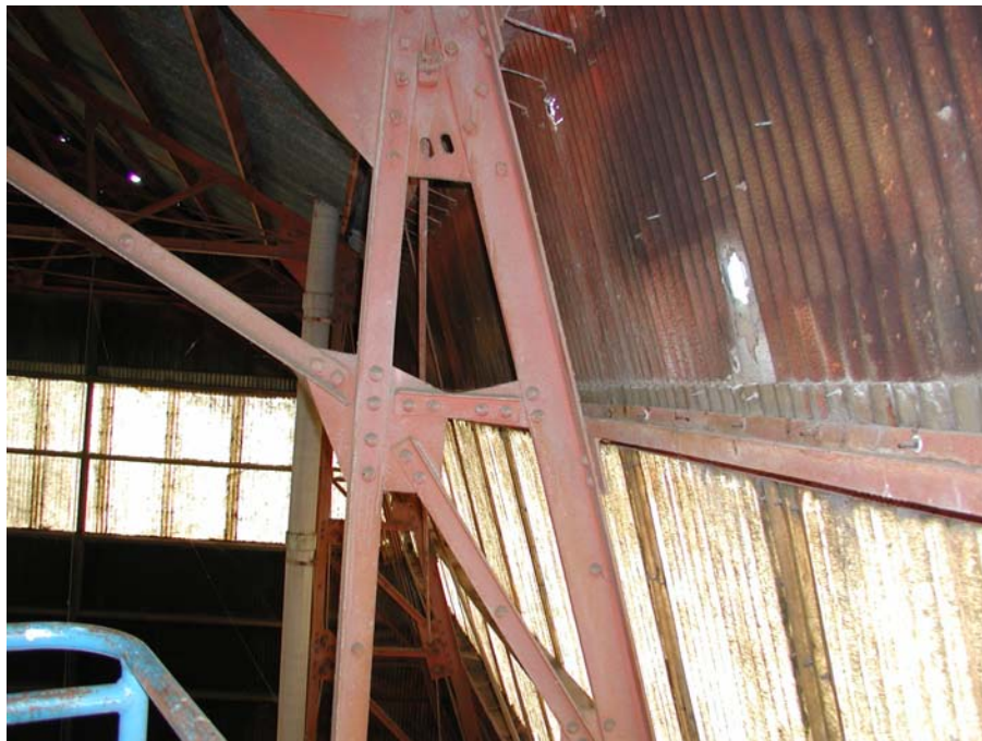
Vertical Truss Gusset Plate
