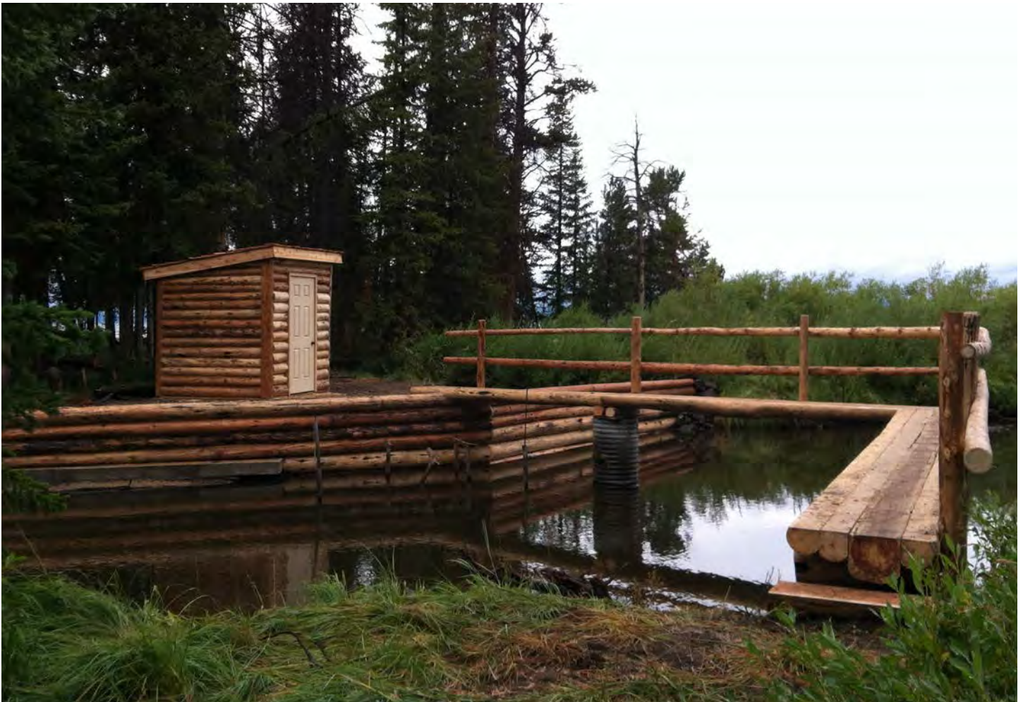
Clear Creek Cutthroat Counting Station, reconstructed in 2012. Spawning cutthroat trout are counted in Clear Creek, a large remote tributary on Yellowstone Lake, using an acoustic monitoring system. -NPS photo
