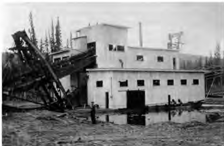
This 1936 photo shows the Coal Creek dredge just before completing construction with the major components in place. The digging ladder and bucket line (left) are in place and the framework for the stacker (right) is beginning to take shape.
