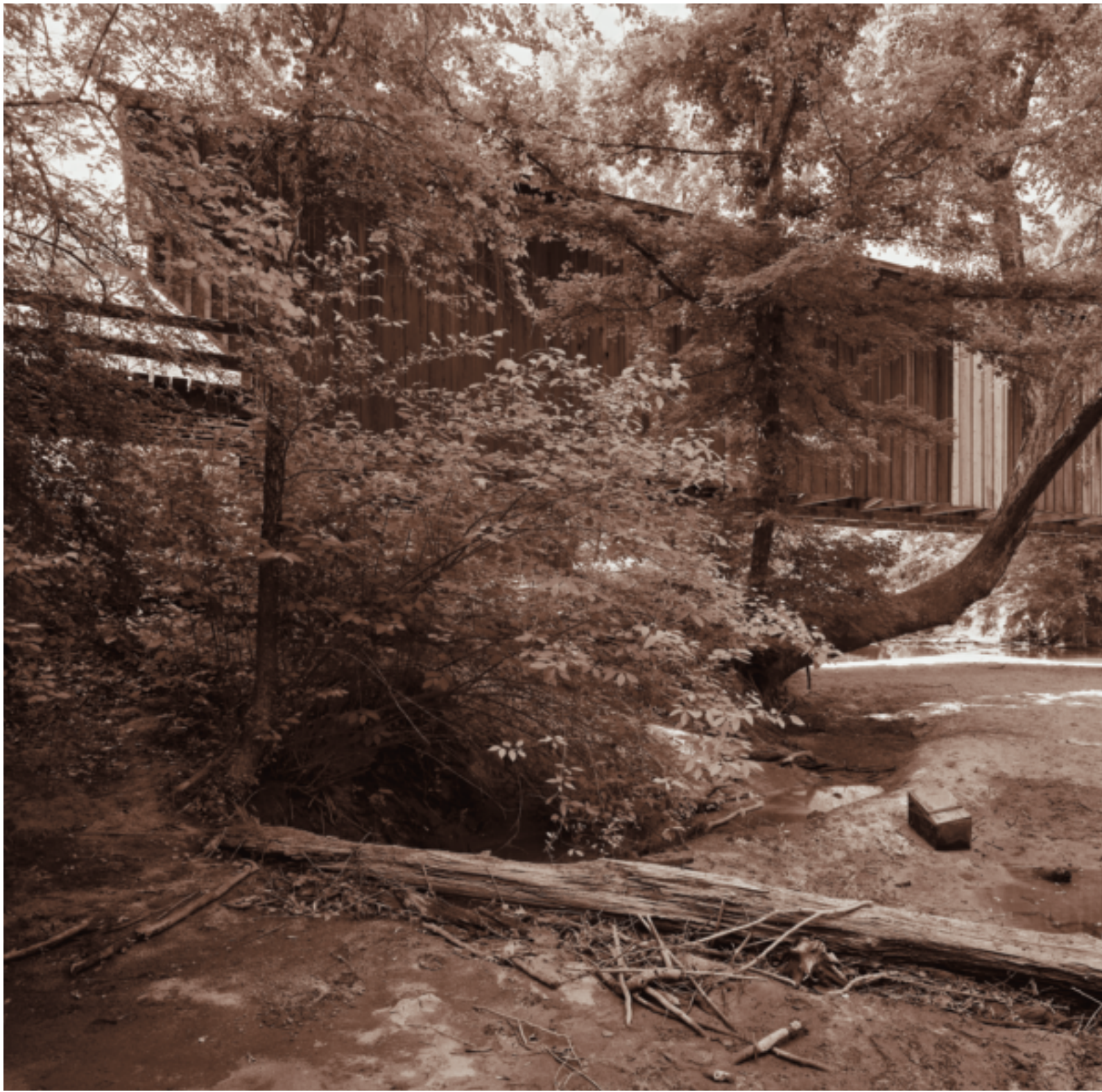
Above: Red Oak Creek Bridge, Merriweather County, Georgia. Rural icons today, covered bridges were 19th-century necessities, the product of a growing population, economic need, and the burgeoning field of engineering and design. This specimen dates from the 1840s.
