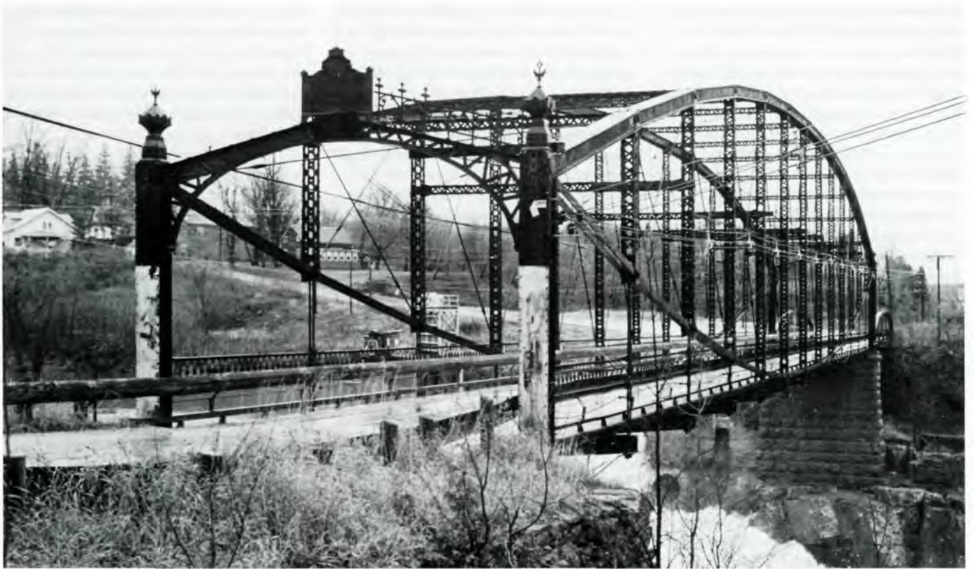
The Douglas and Jarvis Patent Parabolic Truss Iron Bridge in Franklin County, Vermont, is one of many structures listed in the National Register of Historic Places because of its engineering significance. (Chester H. Liebs)
