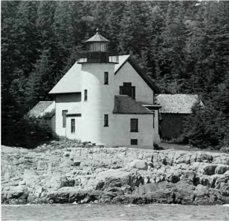
Narraguagus Light Station, near Milbridge, Maine, was surveyed by the State as part of a thematic group of lighthouses and listed in the National Register of Historic Places. (Tom Goettel)
