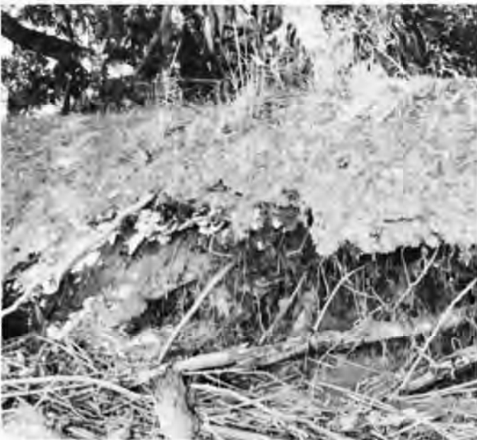
Photo 4 - Bank erosion at CUIS-24.
