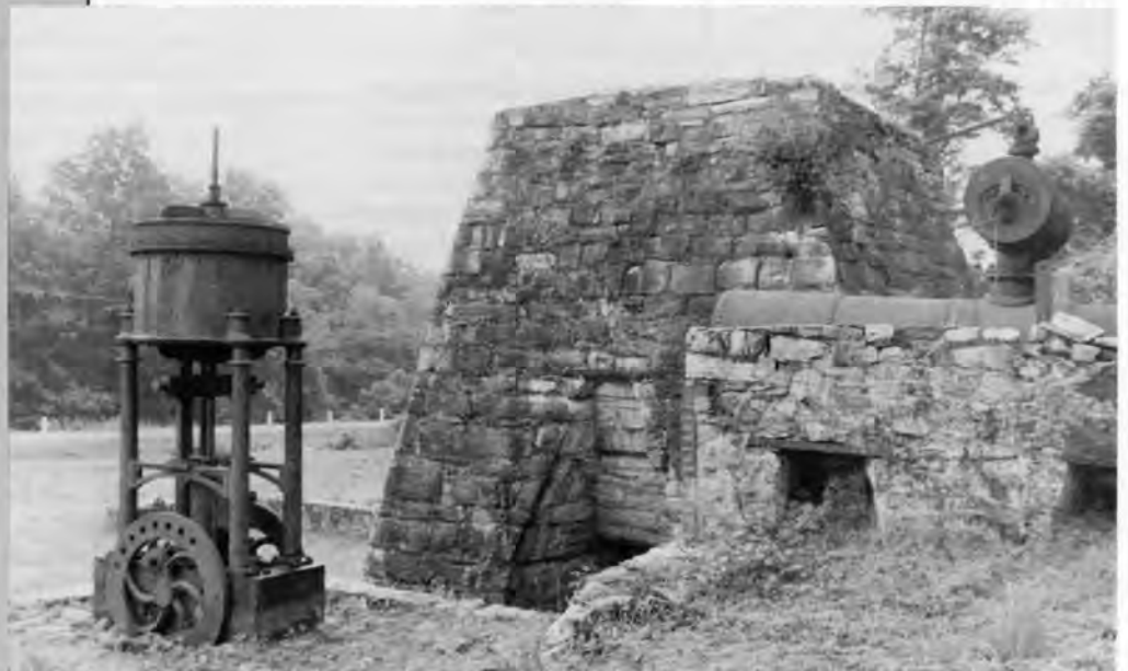
Carrick Furnace, with the blowing engine to the left, the iron furnace stack in the middle, and the boilers to the right. Photo by Diane Reed, Pennsylvania Historical and Museum Commission, 1990.
