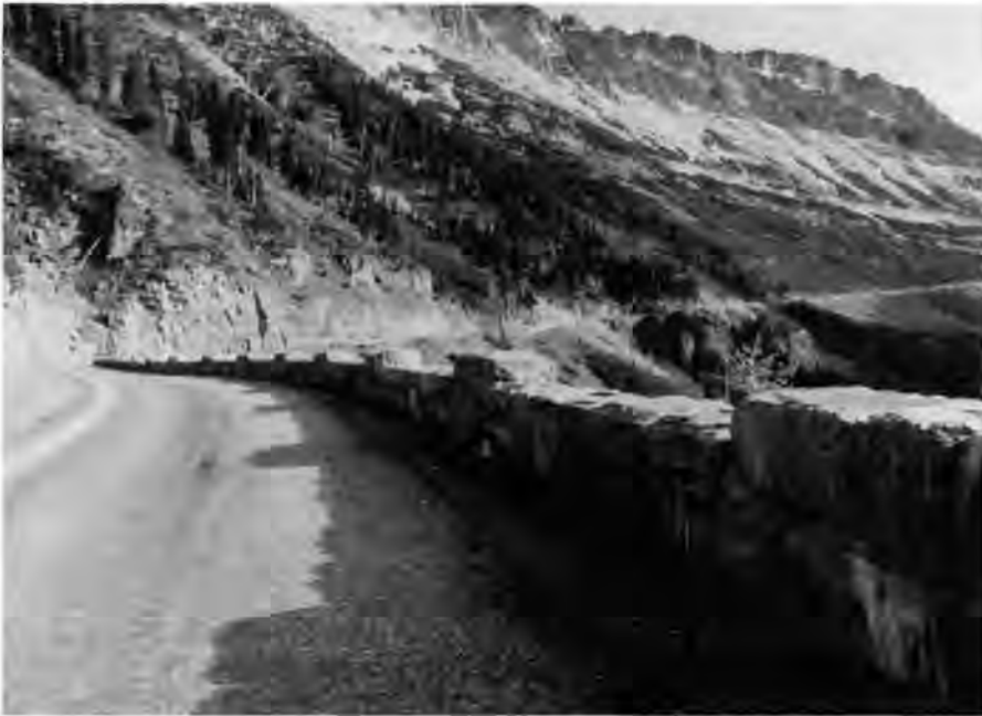
Typical masonry guardwall.
