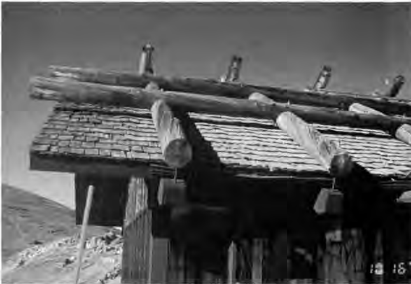
Figure 1 The log snow guards on the Rocky Mountain National Park visitors' center allow snow to accumulate without introducing further stresses to the roof system.
