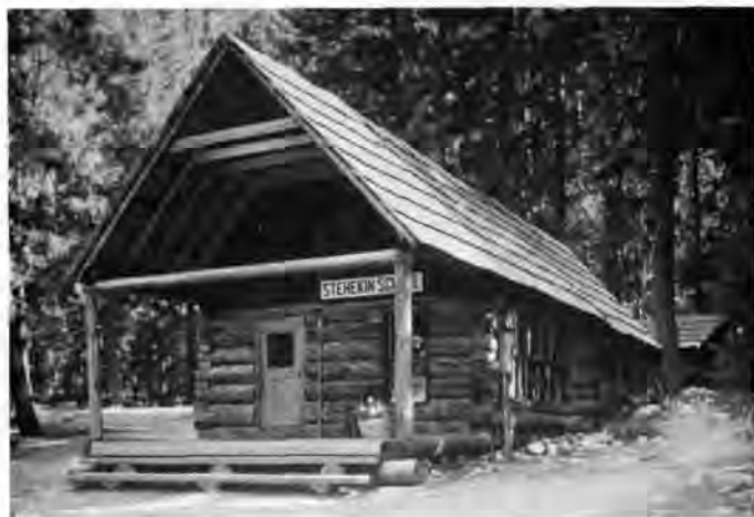
Figure 2 In the North Cascades, a distinct style of cabin has evolved that allows both light and people to enter a snow bound building.
