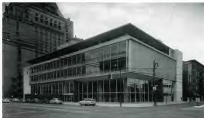
Vancouver Public Library. Semmens and Simpson, 1956-57. Clad in a glass and aluminum curtain wall, the Library's innovative design includes wide column spacing to allow for flexibility and future expansion. Courtesy of Vancouver Public Library.
