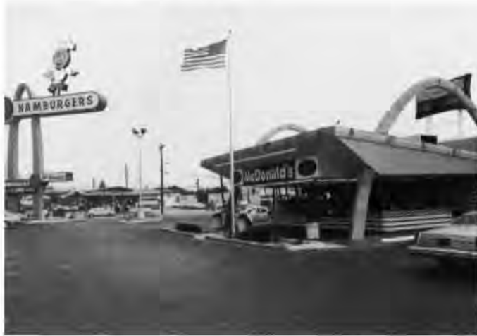
The 1953 McDonald's Drive-in Restaurant and Sign, located on Lakewood Boulevard in Downey, CA, was determined eligible for listing in the National Register on January 19, 1984, as an extremely rare example of its type. The sign, an important part of the property's historic corporate imagery, was threatened by a local ordinance shortly after it was determined eligible. The property is also a designated local landmark. Photo by Alan Hess, 1983.
