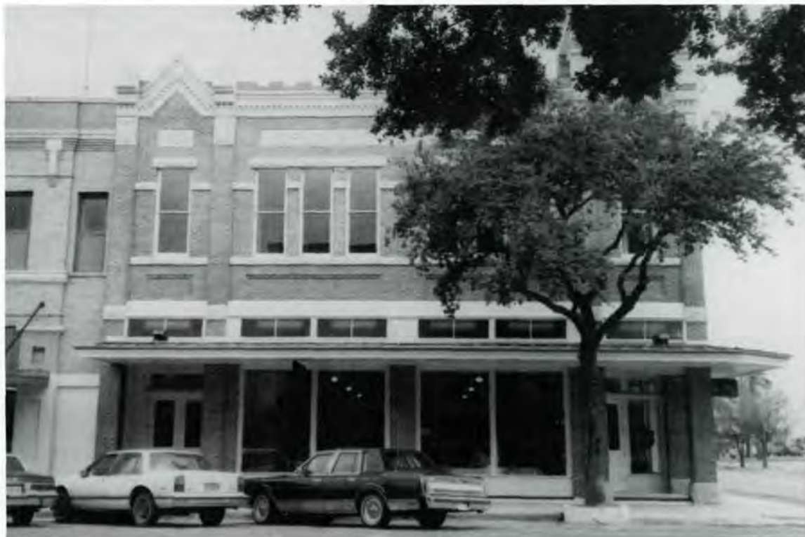
"The Raglands" after the 1989 rehabilitation. Reconstruction of the corner tower (at right) and the first floor storefronts was based on pre-1950 historic photographs. Courtesy of the Texas Historical Commission.
