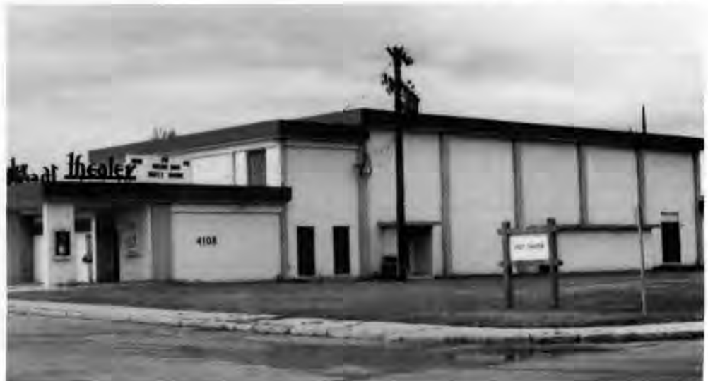
Theater, Fort Wainwright, AK. Built in the 1950s, this theater illustrates a building type designed to improve quality of life on installations for military personnel and their families. Photo by Elizabeth Calvit.
