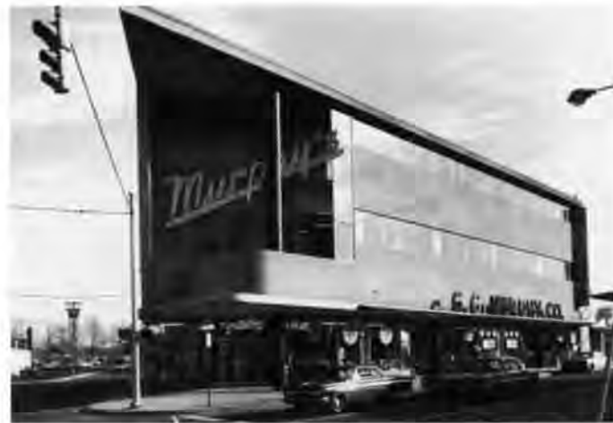
C. G. Murphy Co., Arlington, VA. James F. Hogan, 1948-49. Demolished, 1988. Photo by the author, 1970.
