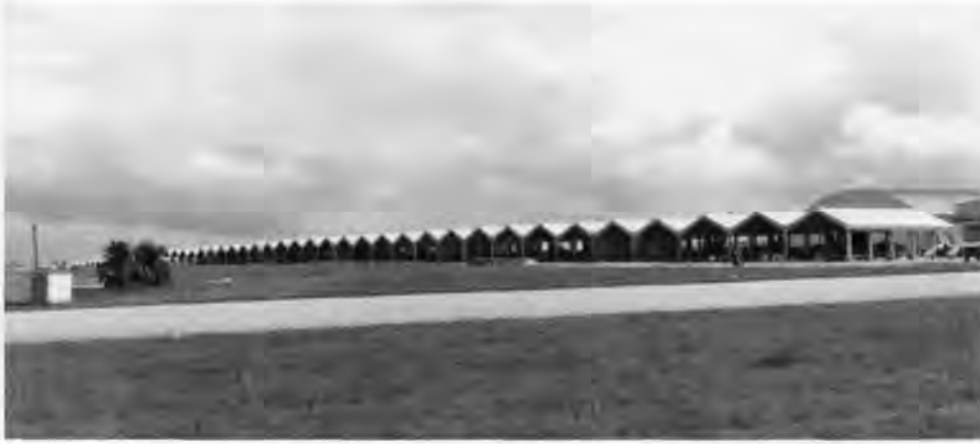
Kadena Air Base, Okinawa, Japan. A product of the Cold War, this unique structure protects aircraft from the elements. More permanent structures shelter aircraft from typhoons. Photo by Elizabeth Calvit.
