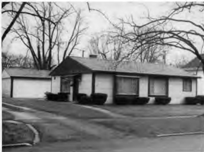
The 1950 Norris and Harriet Coombs Lustron House (and its contributing garage), located in Chesterton, IN, was entered in the National Register on September 17, 1992, as an exceptionally pristine example of the mass-produced Lustron porcelain enameled steel house. Shown are the exterior (above) and an interior view of the bedroom vanity and closet (below) of what has been called the "all-metal dream house." Courtesy of the National Register of Historic Places.
