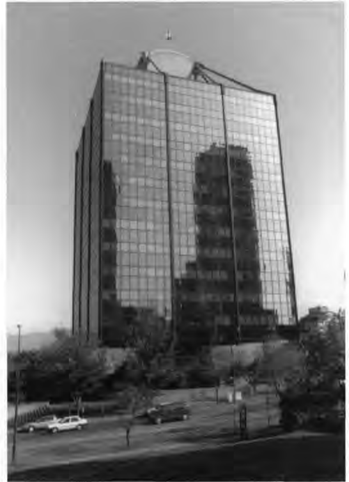
West Coast Transmission Building. Rhone and Iredale with Bogue Babicki, Engineer, 1968-69. One of the first buildings in the world to employ suspension bridge techniques for structural support: a central concrete service core serves as the main structural support; the floors are suspended by thin, continuous steel cables hung from the core. The design also allows for a column-free parking garage and open plaza areas at the building's base. Photo by Marco D'Agostini.
