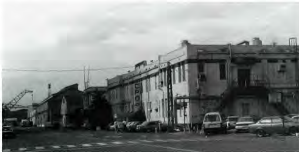
Yokosuka Naval Base, Japan. Main street with its typical installation support buildings — worthy of documentation and, possibly, preservation. Photo by Elizabeth Calvit.
