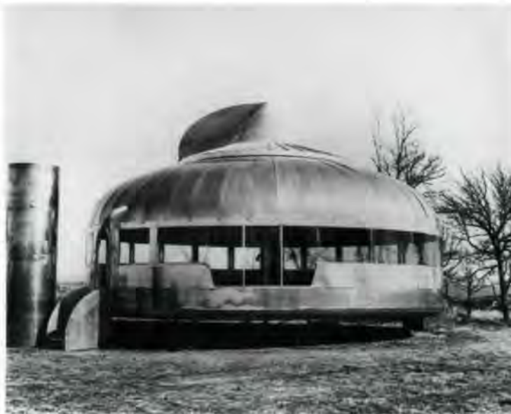
Buckminster Fuller’s Dymaxion House prototype was recently acquired by the museum. The house, seen here as first erected in 1945, was manufactured by Beech Aircraft Corp. of Wichita, KS. Its compact aluminum pieces could be shipped in the returnable stainless steel cylinder at the left. Courtesy of Buckminster Fuller Institute.
