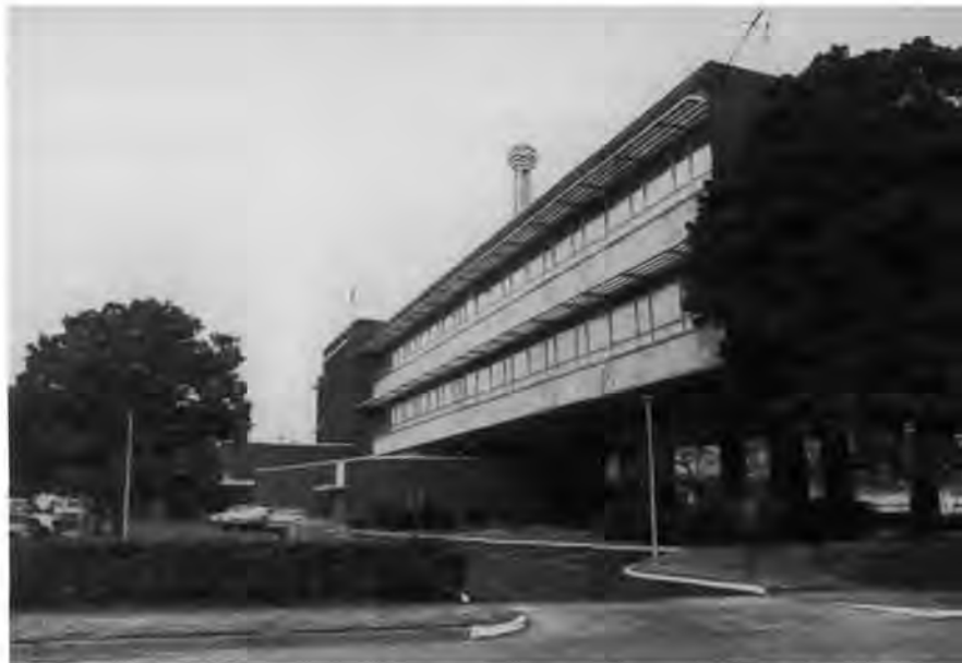
Designed by Fred Arnold and the architectural firm of Wittenberg, Deloney and Davidson, the Arkansas Power & Light Building in Little Rock was constructed between 1955 and 1959. This is an exceptionally notable, virtually unaltered local example of International style architecture and was listed in the National Register on September 14, 1992. Photo by Ken Story, 1992.
