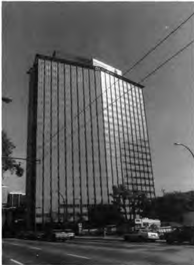
B. C. Hydro Building, Thompson, Berwick and Pratt, 1955-57. The distinctive lozenge shaped building represents a West Coast interpretation of the International Style. Photo by Marco D'Agostini.
