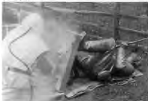
7. J. K. Ellicott, 1st Pennsylvania Cavalry Monument, 1890, bronze and granite, detail. Hancock Avenue, GNMP. Photograph depicts bronze figure being cleaned to bare metal using glass bead peening in 1979. Photo courtesy of GNMP.
