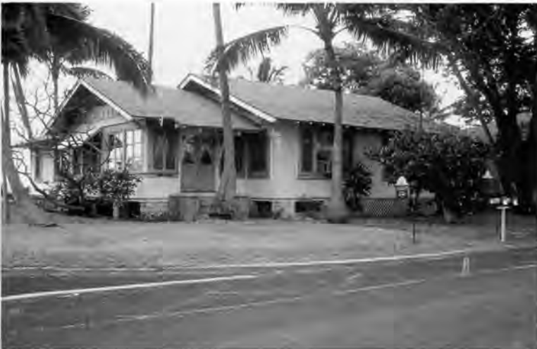
Single-wall, wood-framed, Hawaiian plantation style houses constructed in 1922.
