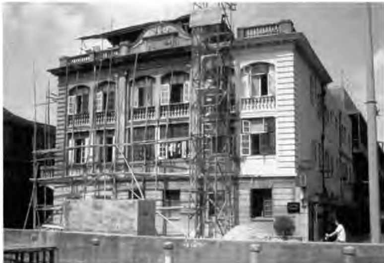
Warehouse being repainted, Shanghai.
