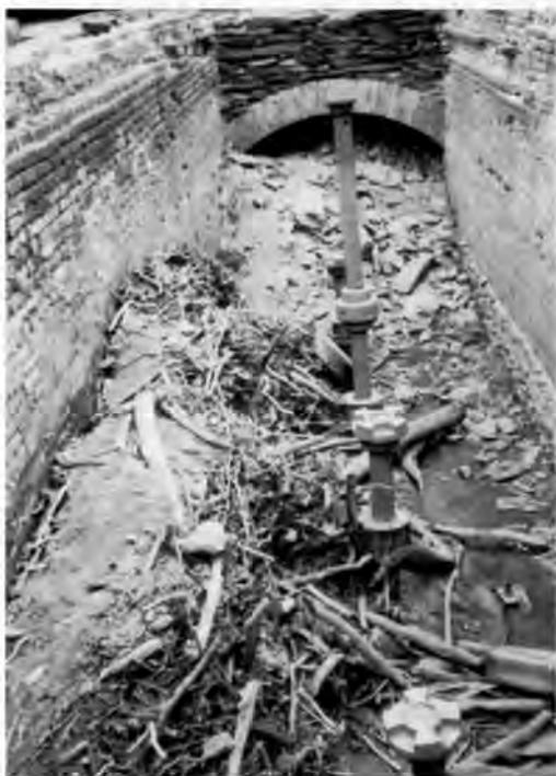
Virginus Island flood damage, 1996. Flood debris and damaged masonry in the turbine pit of the cotton/flour mill ruins.
