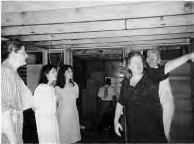
Preservation work was explained during the construction process at Pope-Leighey House, Mt. Vernon, Virginia (Woodlawn Plantation). Good job site tours, which require a collaboration with the contractors and artisans, are always popular as well as educational. Photo by the author.
