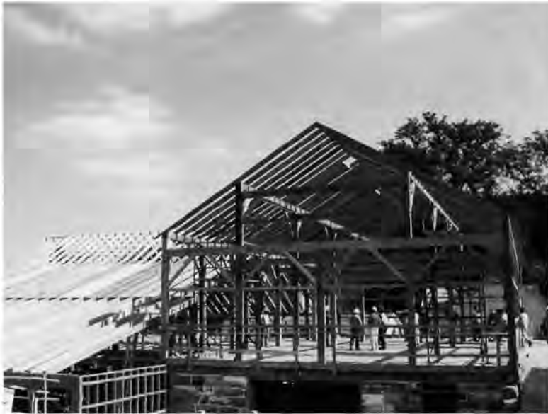
Completed timber frame at main dairy barn, Malabar Farms State Park.
