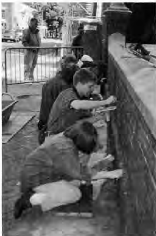
Nick Wyman, assistant park historical architect, and Lenette Curtis, architecture intern, learning masonry skills at a brick repointing workshop at Independence National Historical Park. Photo by the author.
