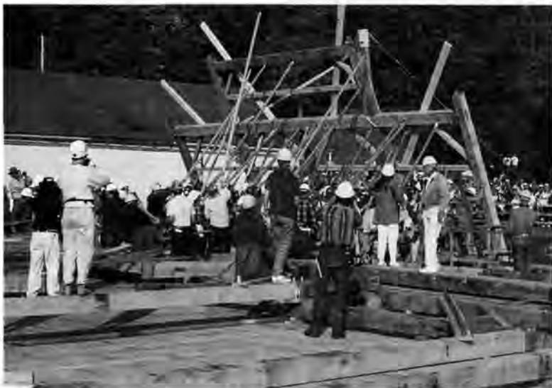
Main dairy barn at Malabar Farms State Park. "Hand raising" of timber frame bent with the help of Ohio Governor Voinovich.
