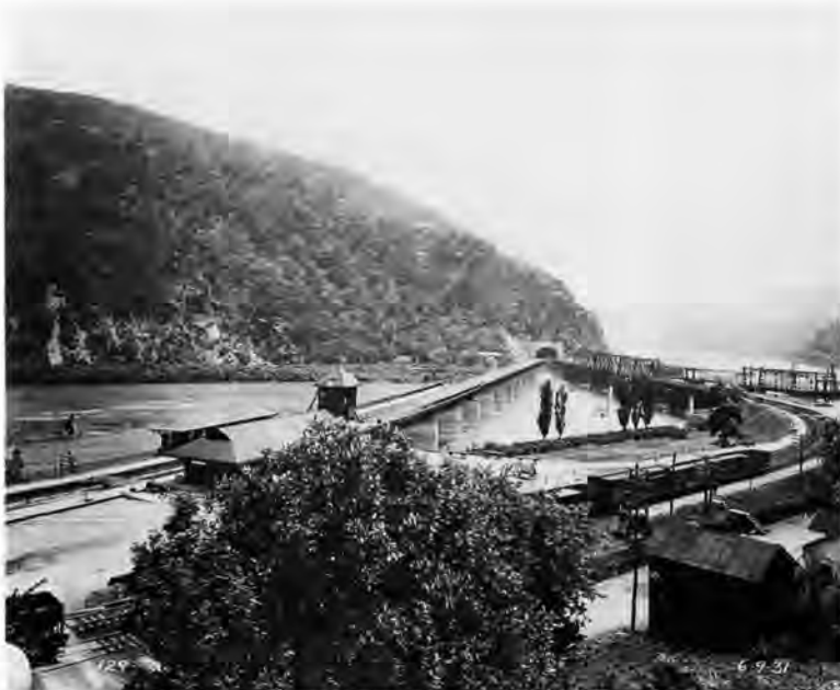
This 1931 photo of B&O bridges at Harpers Ferry (1868 iron Bollman truss partially hidden at right, 1894 steel Pratt truss at center, 1931 steel deck-girder at left) depicts three distinct eras in U.S. bridge building technology. Photo courtesy NPS.
