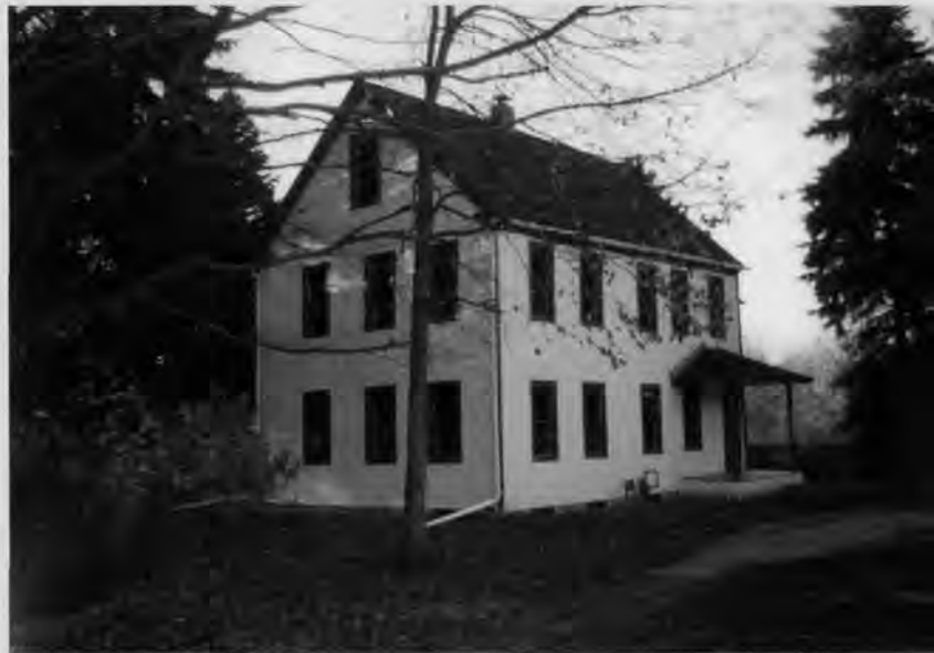
S & H Wiesneans House. Constructed, 1915; Boston Mills Historic District.
