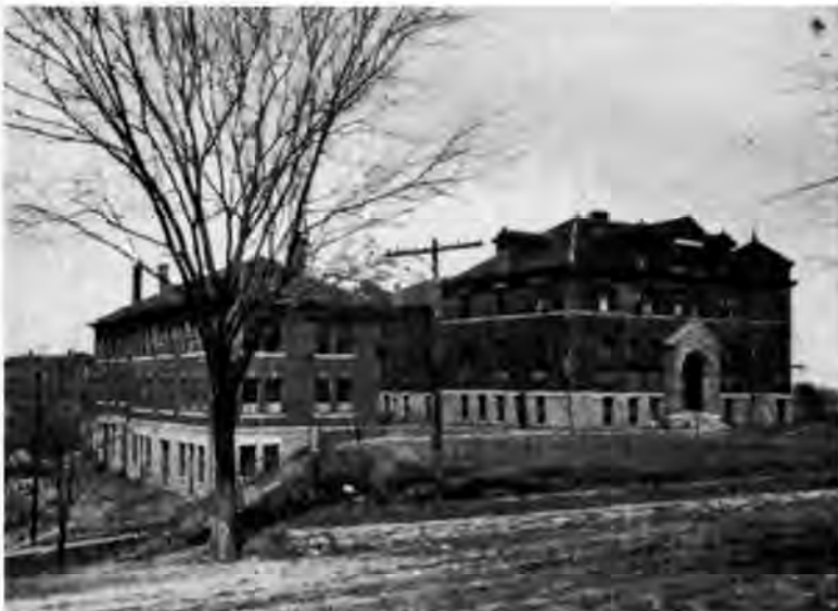
One of the buildings of Western (Freedmans) University overlooking Quindaro, 1920s. Photo courtesy Kansas State Historical Society.
