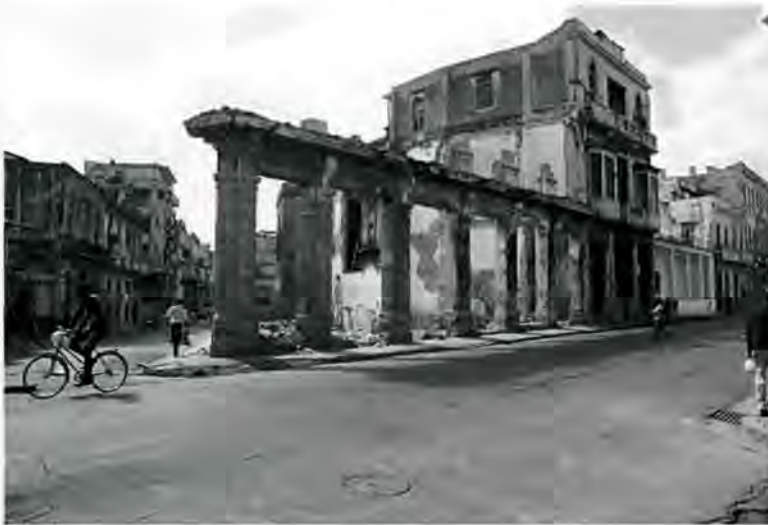
Remains of a collapsed building near the Malecon, Havana, Cuba. Photo by the author.
