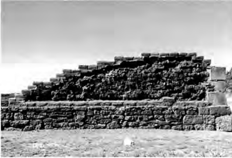
Forge House, Fort Davis National Historic Site (north elevation, north wall).
