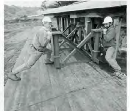
Jim Matyiko and Richie Meekins of Expert House Movers install temporary support system. Photo by Mike Booher.
