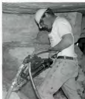
Mike Vakanti removes foundation stones before the lighthouse can be lifted from its present foundation. Photo by Mike Booher.
