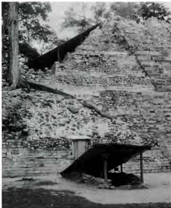
Copán, Honduras. Structure 16 showing tunnel access to excavation areas.
