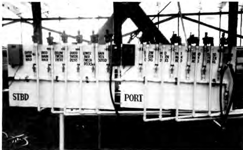
Three times a day, an intricate system of tubes and valves sprays an aqueous solution on the interior of Wapama to arrest her most serious ongoing problem — dry rot decay. Photo courtesy of National Park Service
