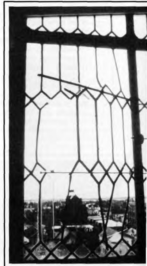
Winds of 140 miles per hour and flying debris destroyed windows throughout the city. The loss of architectural details found in such elements as this leaded-glass window—major long-term effect of Hurricane Hugo. Photo by NPS.
