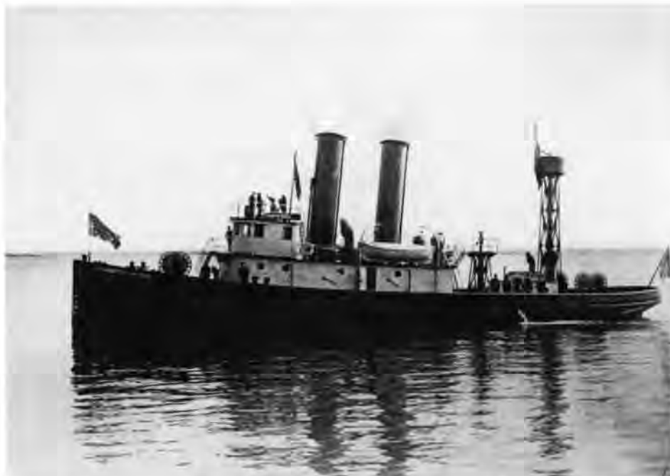
City of Philadelphia Fireboat "J. Hampton Moore," equipped with Babcock & Wilcox boilers.
