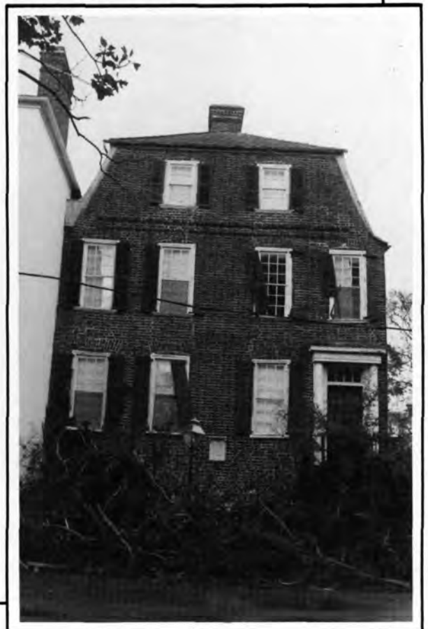
Exterior facades took the brunt of hurricane winds. In many instances, shutters which could not be closed because of poor maintenance were severely damaged by the storm. Photo by WPTC, NPS.
