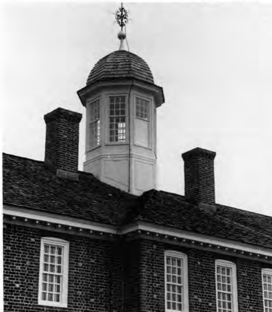
Pressure-impregnated fire-retardant cypress shingles were installed on the reconstructed mental hospital at Colonial Williamsburg. Photo by Rudd M. Long.
