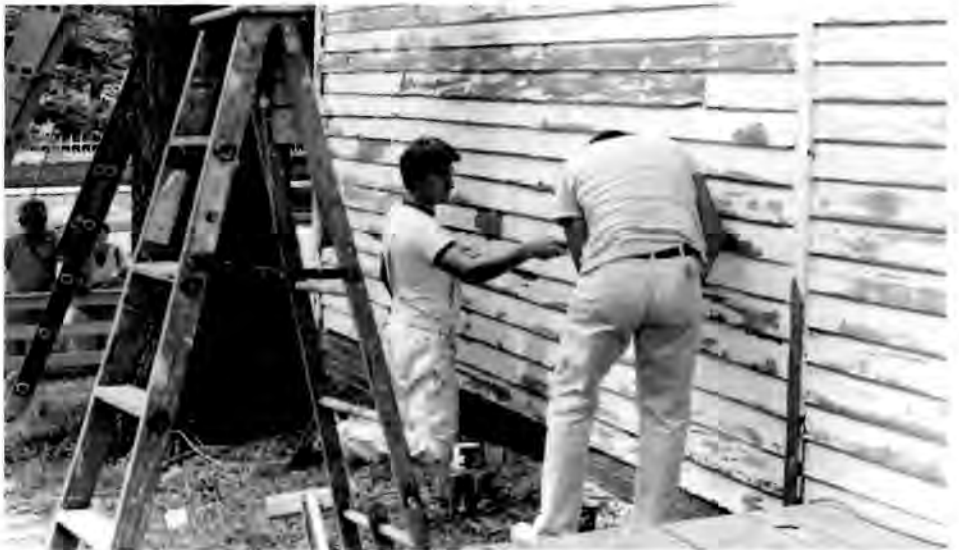
Workmen prepare the Corneau House for the Historic Leasing Program.
