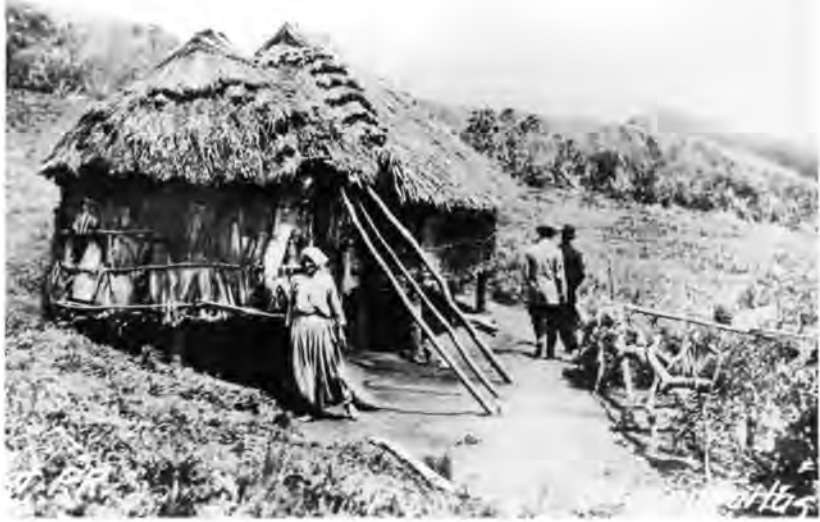
FIGURE 3 Changes in the original Puerto Rican bohío type are evident here. A second unit next to the original one was a common solution to the needs of a growing family. (Unknown source, 1916.)
