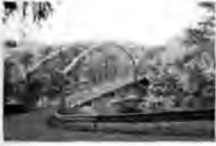
FIGURE 4 This uncommon multiple-span lenticular truss bridge carries Dutchtown Road over the Susquehanna River in Broome County and is listed in the National Register. (Courtesy of Mead & Hunt, Inc.)
