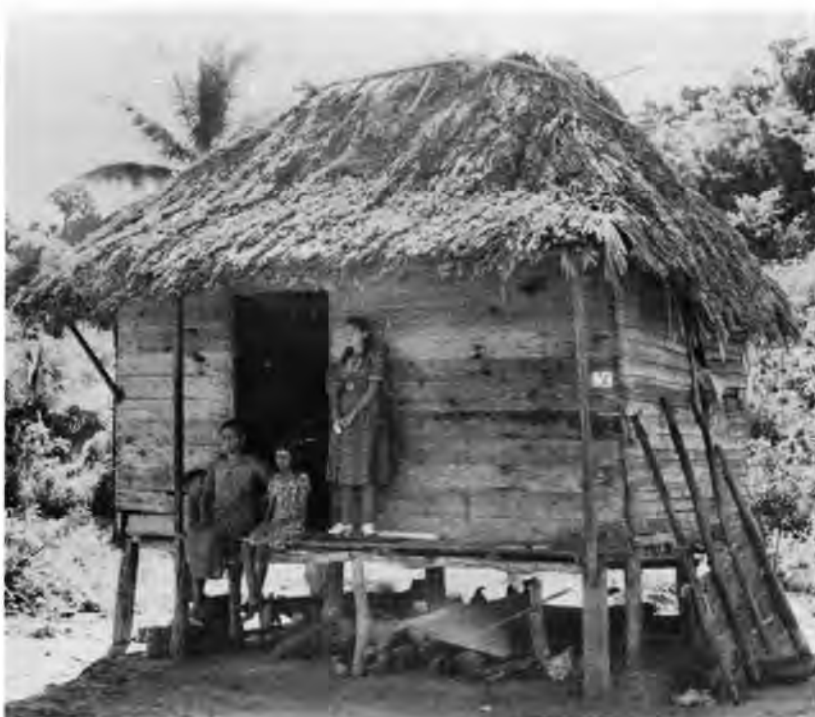
FIGURE 5 Another example of an evolved bohío, using wooden planks obtained from the palm tree ( tabla de costa or tabla de palma ). Notice the ramp-like artifact seen at the right of the image. (Unknown source, circa 1930-1940.)
