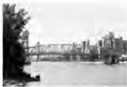
FIGURE 1 The Roosevelt Island Bridge over the East River in New York City is an example of a vertical lift bridge. (Courtesy of Mead & Hunt, Inc.)
