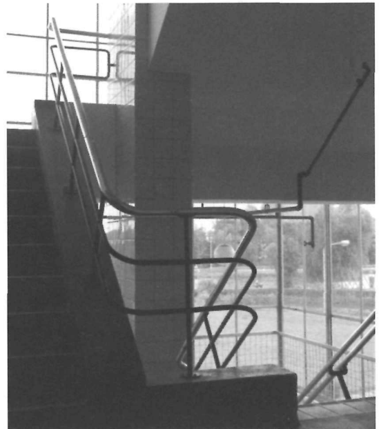
FIGURE 6 Restored interior stair.
