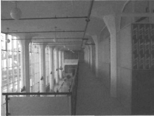
FIGURE 3 Interior with internal glass enclosures.
