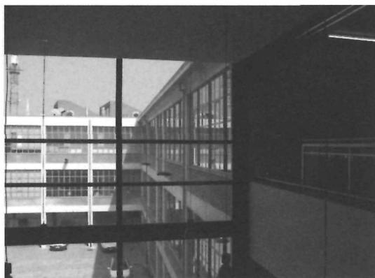
FIGURE 9 Interior of addition looking into courtyard.
