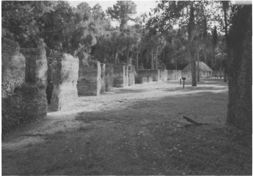
FIGURE 3 Kingsley Plantation slave cabin structures, view looking southeast along the east range of slave quarters. HABS FL-478-21 (Jack E. Boucher, photographer, September 2003. Courtesy of the Historic American Buildings Survey, National Park Service)
