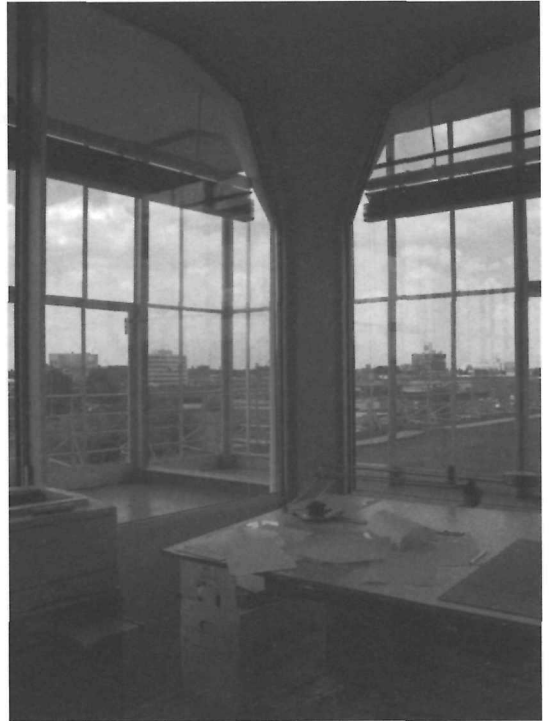
FIGURE 5 Office; view out through interior glazing and curtain wall.
