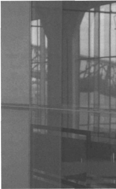
FIGURE 4 Detail of new interior glazing.
