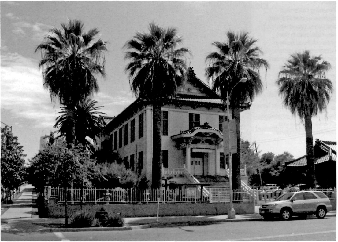
FIGURE 2 Fresno's grand Buddhist temple was built in 1920 after a fire destroyed the original 1902 structure. Preserving California's Japantowns surveys found a relatively large number of extant buildings that represent the heart of most Japantowns: Christian churches, Buddhist temples, community halls, and Japanese language schools. These structures were the primary places for Japanese immigrants and their children to gather as a community and preserve traditional cultural practices. (Courtesy of Preserving California's Japantowns )
