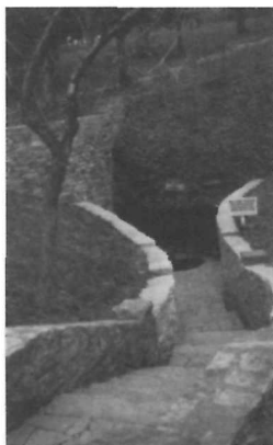
FIGURE 5 The U.S. War Department built the steps and retaining walls shown in this 1934 photograph to facilitate public access to the Sinking Spring. (Courtesy of the National Park Service)
