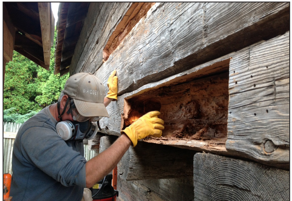
A Coupeville Lion removes rot during a restoration grant project on the 1855 Alexander Blockhouse
