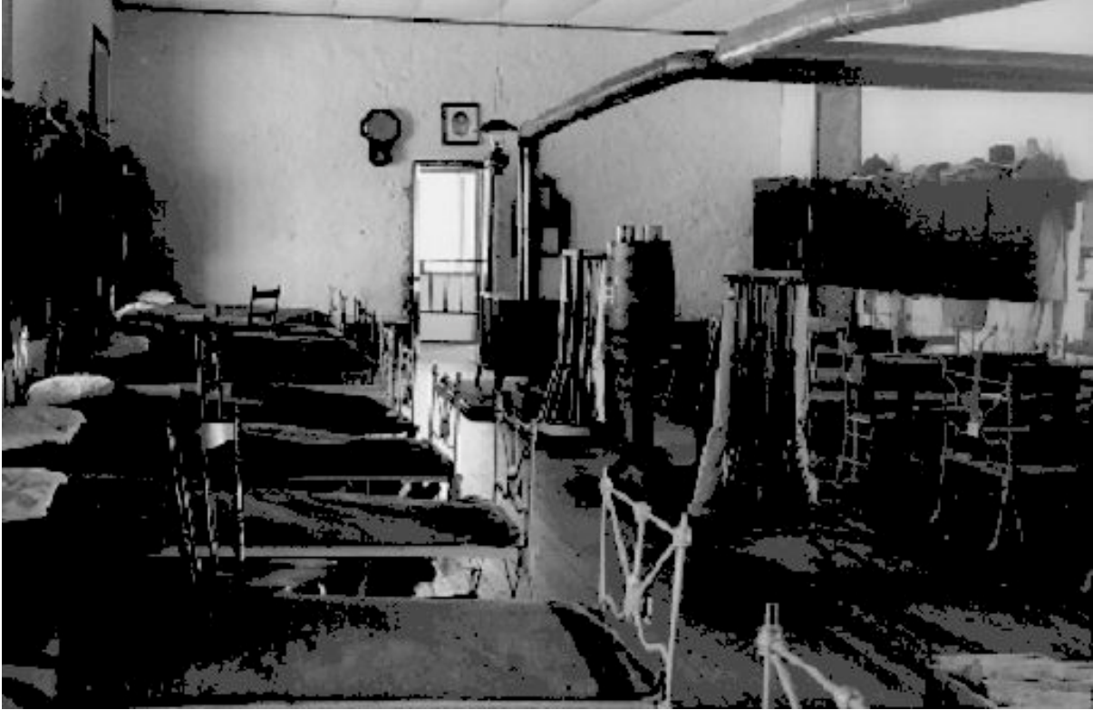
Squad Room of Refurnished Enlisted Men's Barracks
