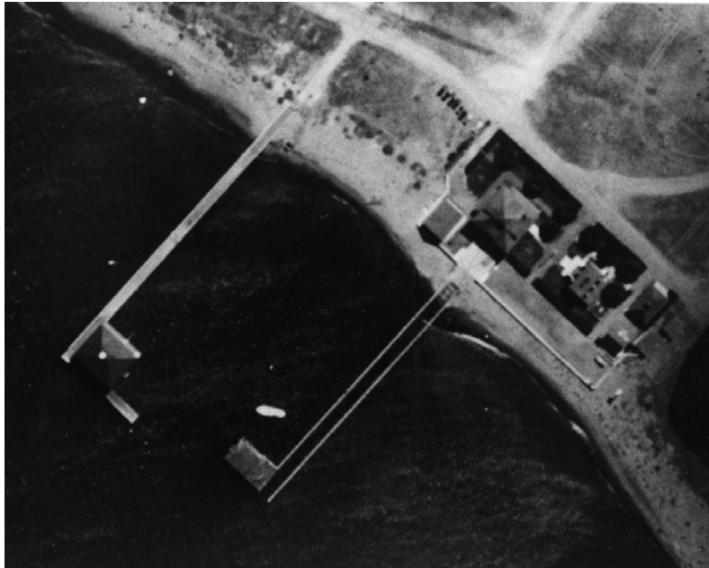
History figure 7. Aerial photograph from about 1938. This view corresponds closely with the site plan drawn up that year. Note that old boathouse (PE 1902) has not yet been aligned with buildings PE 1901 and PE 1903. Maintenance shop (PE 1907) at head of marine railway shows original north-south orientation of roof. [34]
