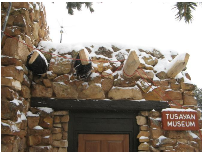
Heating pads over the viga ends
