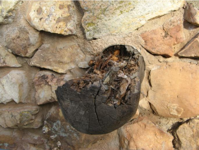
Viga ends prior to preservation
