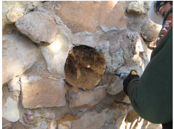
Removing rotted viga end
