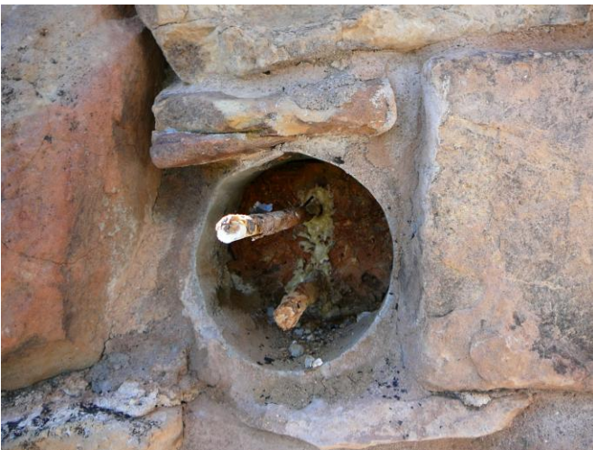
Borate impregnated rods
