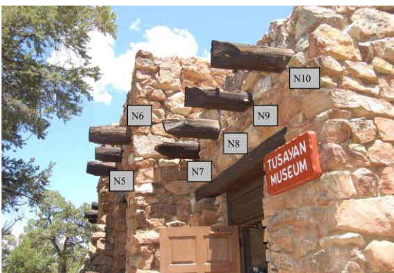
North Elevation Vigas
