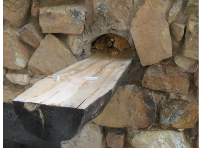
Dutchman half log repair in progress
