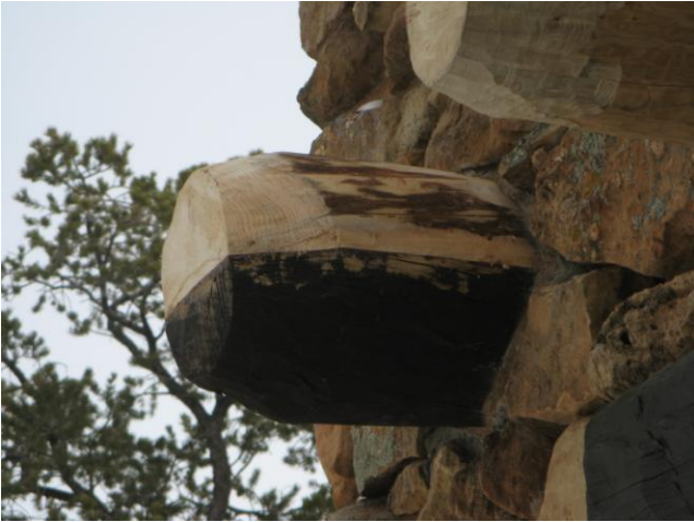
Dutchman half log repair, rounded end
