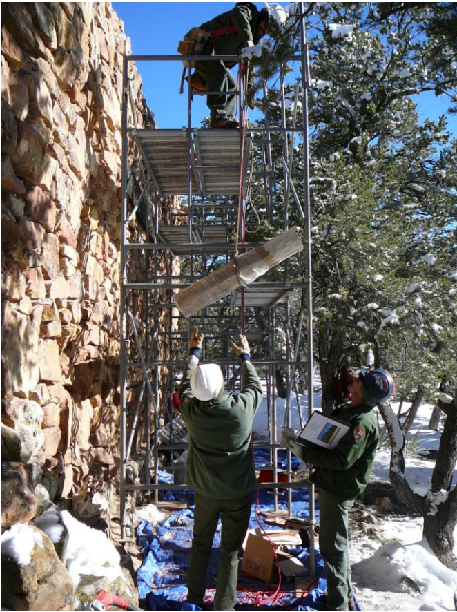
Raising viga end replacements
