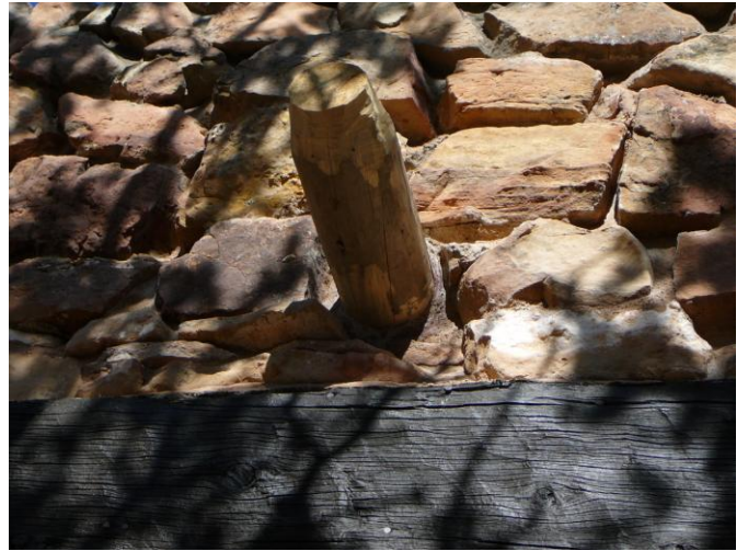
Complete replacement, rounded end
